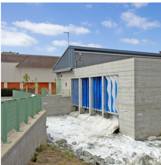
The San Francisquito Creek Storm Water Pump Station installed in 2009 clears storm water from streets in a 1,250 acre neighborhood in northeastern Palo Alto.
