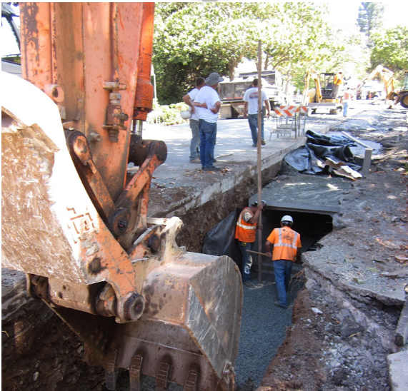
New storm drain pipes were installed along Channing Avenue in 2011 to reduce frequent street flooding along this important vehicle and bike corridor.
