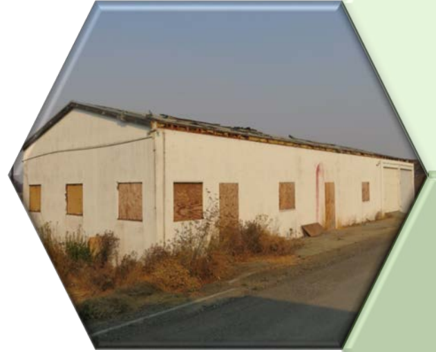
ITT office building before deconstruction.
