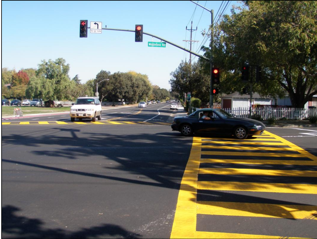
Photo 1: View NE along East Meadow Dr. from the intersection with Middlefield Rd.
