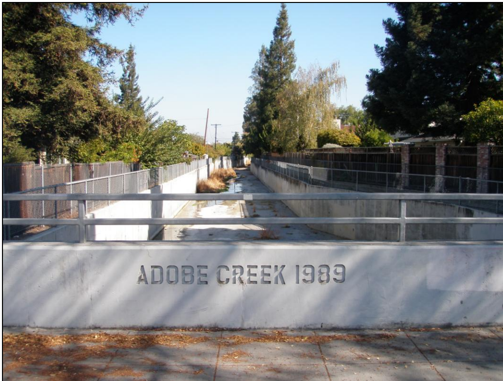
Photo 12: View SW along Adobe Creek at the Middlefield Rd. crossing.
