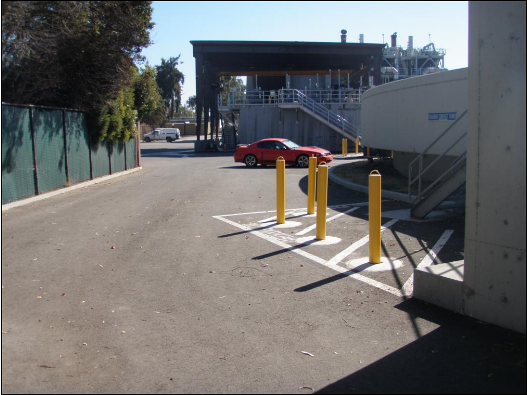
Photo 19: View SE inside the RWQCP at another possible location for tanks.
