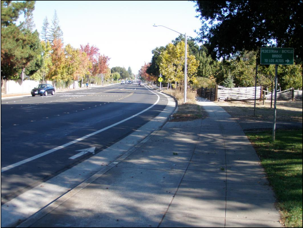
Photo 10: View NE along Arastradero Rd. from Miranda Ave.
