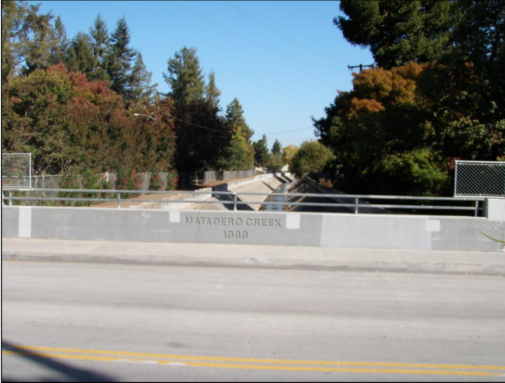
Photo 4: View NE along Matadero Creek at the Cowper Street crossing.
