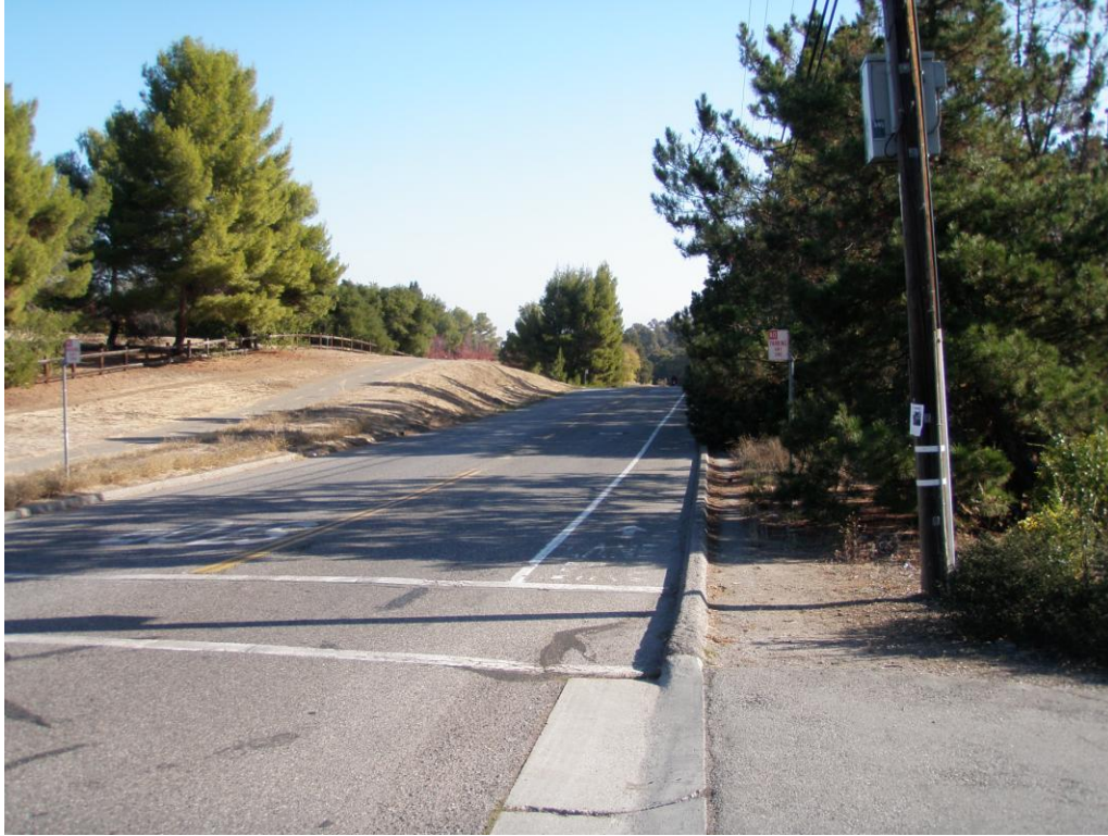
Photo 11: View NE along lateral from Deer Creek Drive to Hillview Ave.
