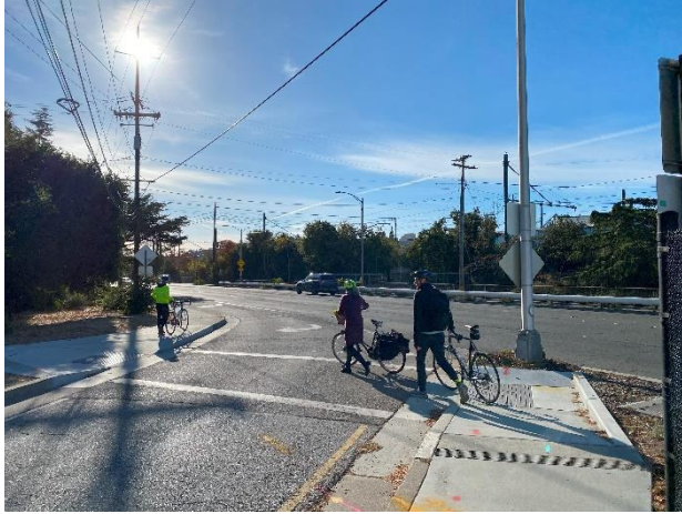
Oregon Expressway on ramp from Alma Street
