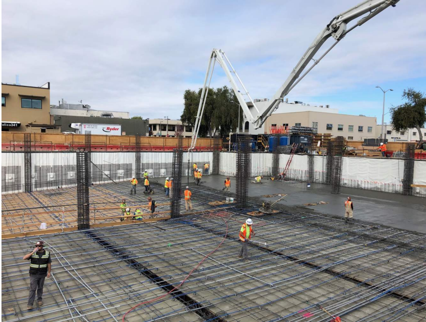
Ramp slab and B1 deck being placed.
