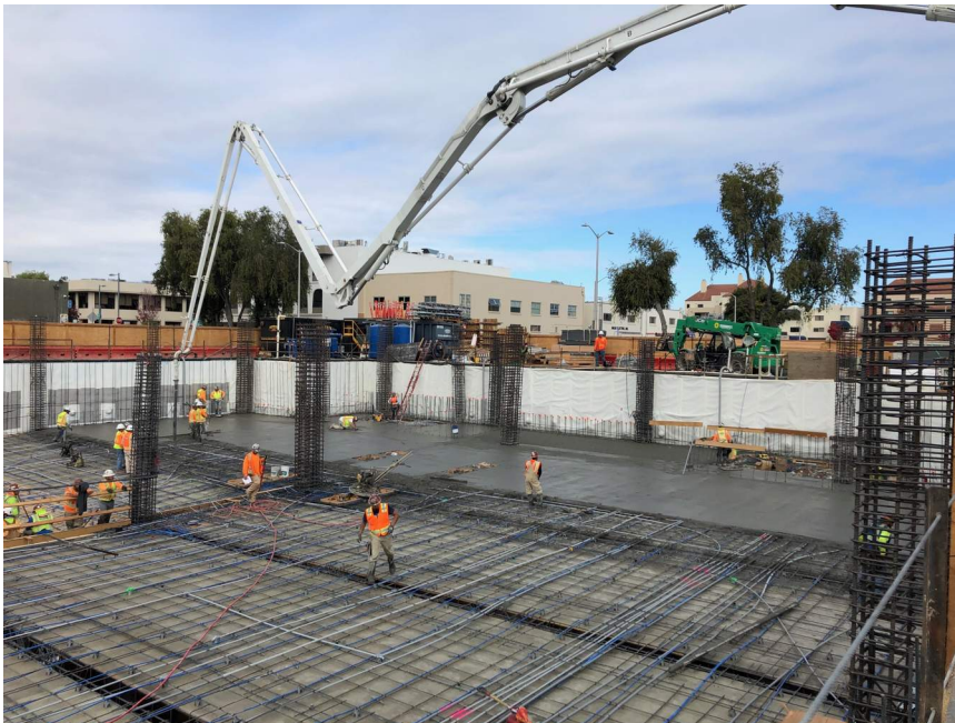
1 st half of B1 deck being placed.
