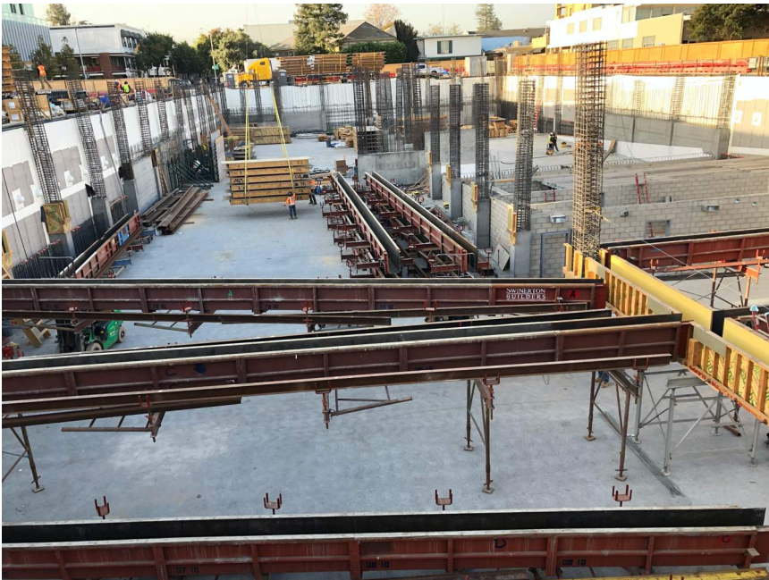
Cunningham beams and table forms being installed for the B1 deck.
