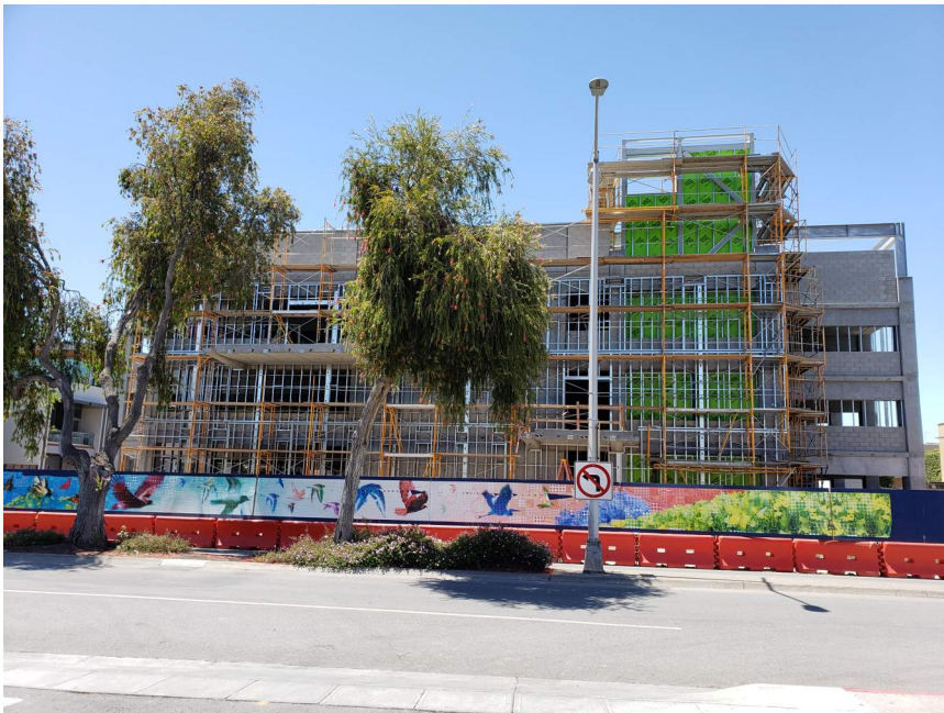
Framing for tile wall ongoing along Birch St. elevation.
