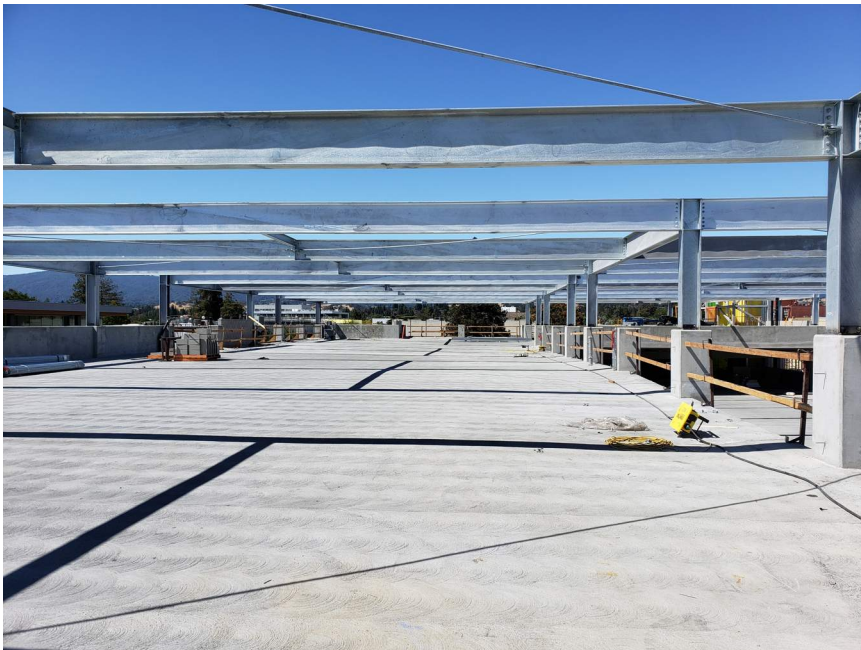
Structural steel for future PV system on roof level.
