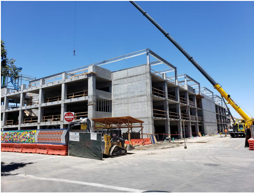
Crane installing steel structure for future PV system.
