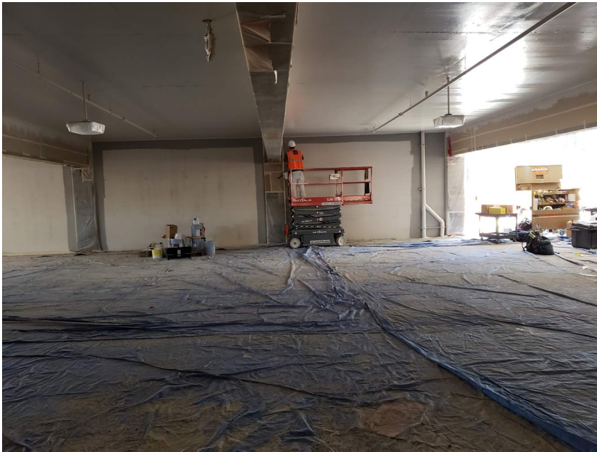
Interior paint ongoing.
