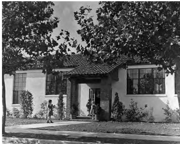
Figure 13: Children's Library, 1940. Source: Palo Alto Historical Association.
