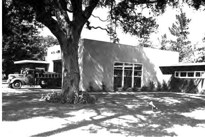
Figure 18: Fire Station No. 3, ca. 1950. Source: Andrew Christensen, Jr., Palo Alto Historical Association.
