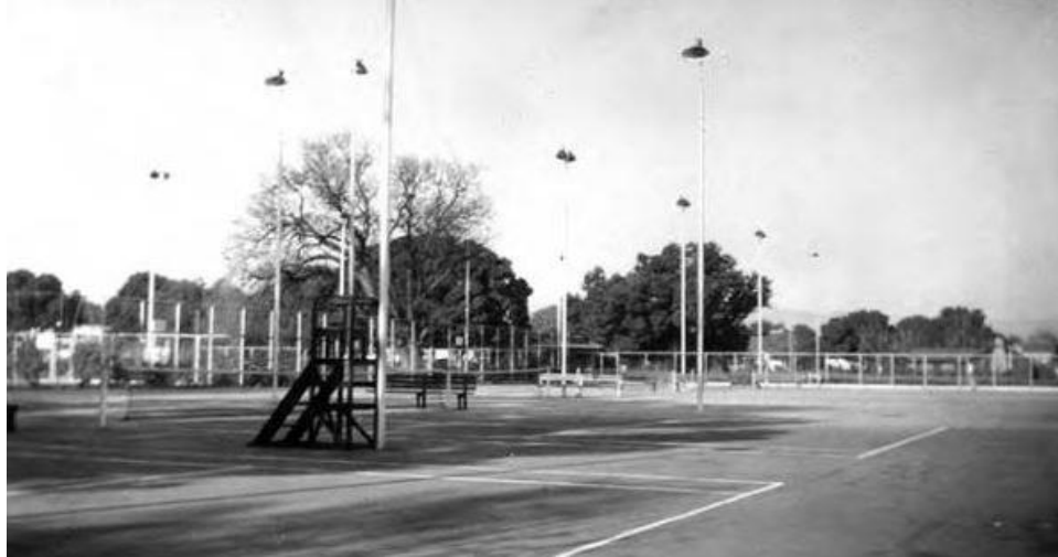
Figure 10: Rinconada Park tennis courts, ca. 1930s. Source: Palo Alto Historical Association.
