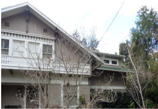
This side addition to an early home in Professorville is visible from the street but is clearly set back from the original front façade.
