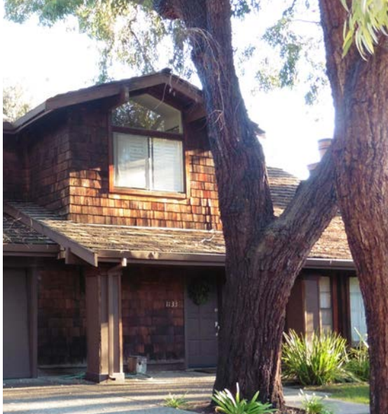
Some newer residences are clad in wood shingles, reflecting Professorville's historic material palette. Retaining these shingles would help to relate homes from different eras within the district.
