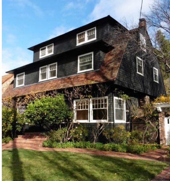
The upper dormer on this home was an early intervention and should not be considered to detract from the overall historic character.
