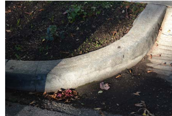
This curb cut with a tight radius reflects an earlier era of Professorville and could serve as a template for future improvements.
