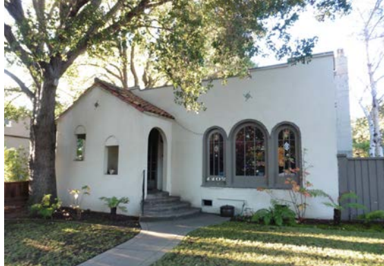
Stucco cladding, tile roofs, and arched openings are characteristic of homes influenced by Spanish Colonial architecture.
