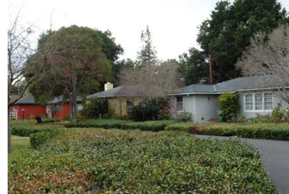
The modest cottages making up Kingsley Court were constructed after the first wave of development of Professorville, but they were designed by Birge Clark, an important Palo Alto architect. Keep in mind that later buildings in the neighborhood may have their own grounds for historic significance.
