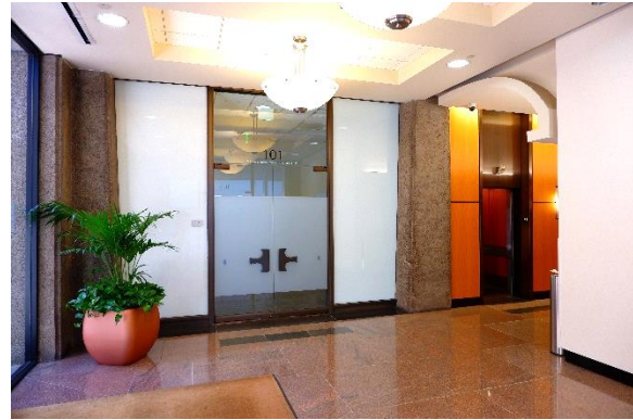
Figure 12. Exposed concrete columns are located in the lobby space. Floor and ceiling materials are non-original.
