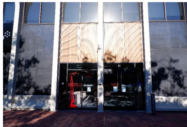
Figure 27. Corrugated metal panels over the doors.
