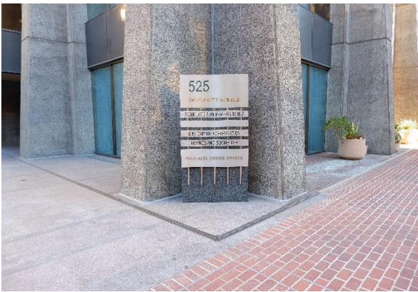
Figure 32. Original brick paving (right) and replacement granite paving (left), with free-standing sign at southeast corner of the Office Tower.
