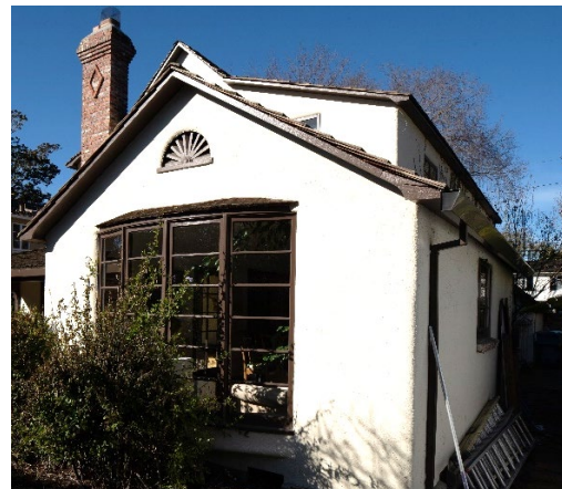
Figure 8: Non-original bow window and rear addition, looking northwest.
