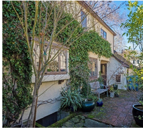
Figure 10: Projecting bay and central portion of the northeast façade, looking north.
