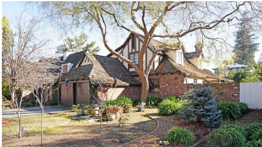
Figure 12: Front yard, looking east.
