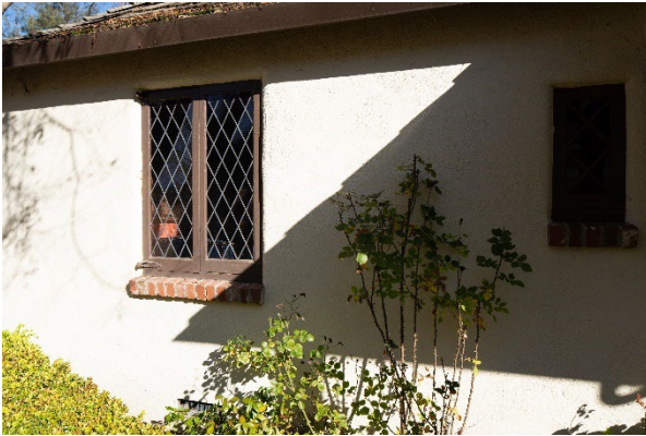
Figure 4: Leaded glass window at the northwest end of the southwest façade.
