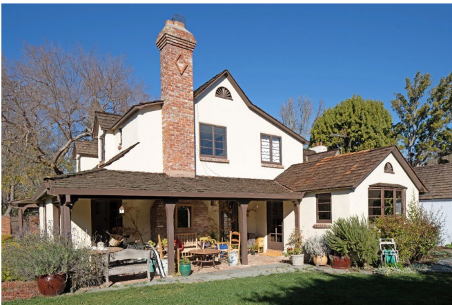
Figure 7: Rear façade, looking north.
