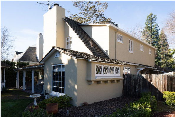
Figure 15: Residence at 534 Santa Rita Avenue, viewed from the side yard, looking west.
