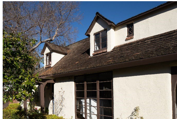
Figure 6: Oblique view of the southwest façade, looking north.
