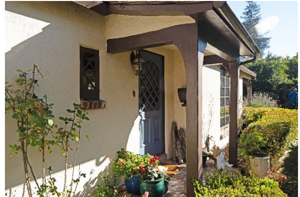
Figure 5: Side entrance at the southwest façade.
