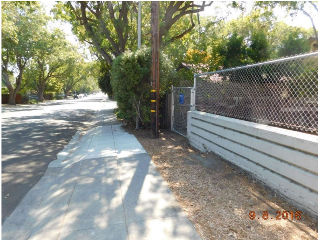
Photo 2: Excessive sidewalk slope and rolled curb, which does not allow for vault placement.
