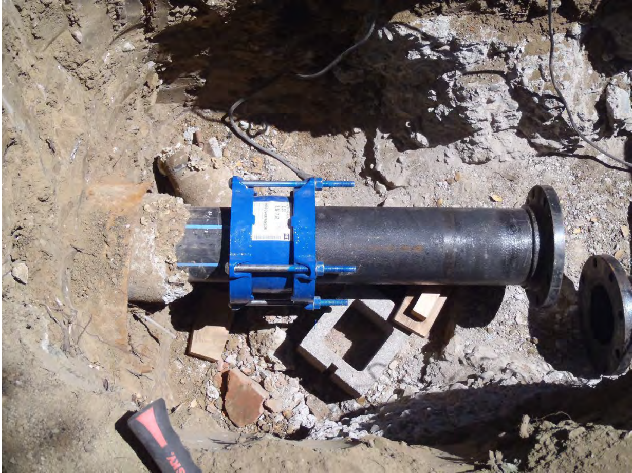
Figure 3-HDPE to DIP Connection with Smith Blair 461 Coupling
