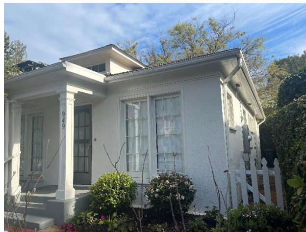
Figure 3: South half of southwest facade.
