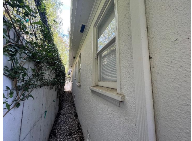
Figure 5: Northwest facade, looking northeast.
