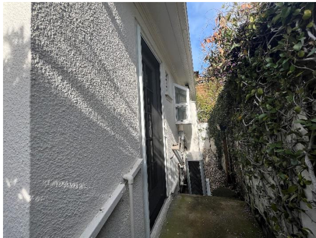
Figure 6: Northeast facade, looking west.
