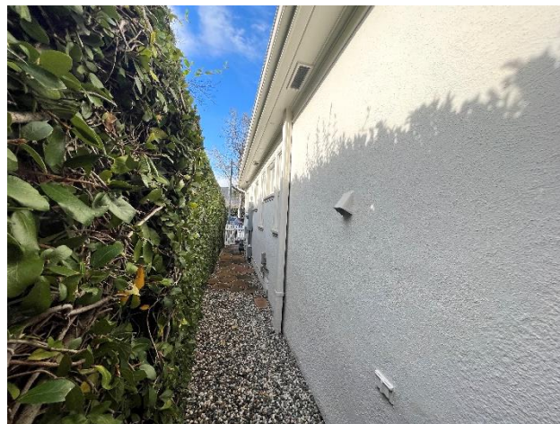
Figure 10: Southeast façade, looking southwest.
