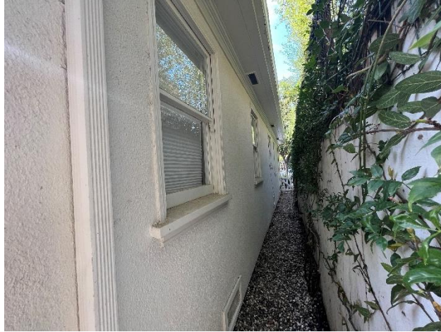
Figure 4: Northwest facade, looking southeast.
