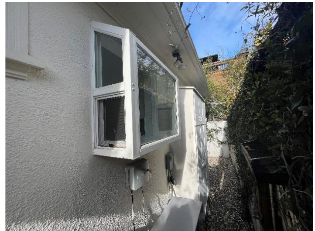
Figure 7: Northeast facade, looking west.
