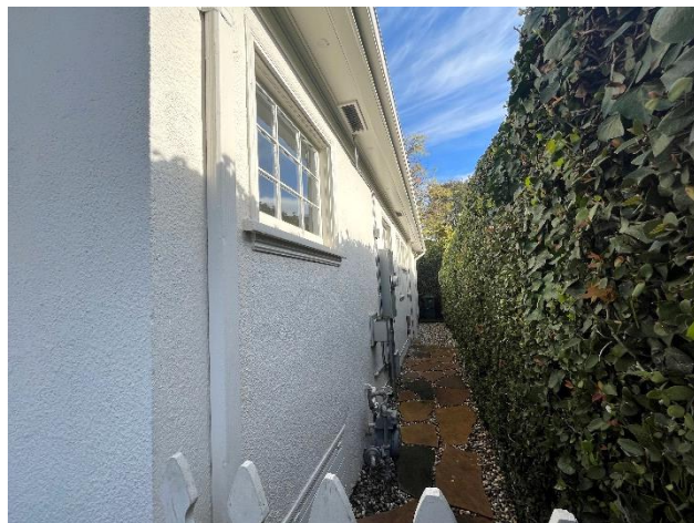
Figure 9: Southeast façade, looking northeast.
