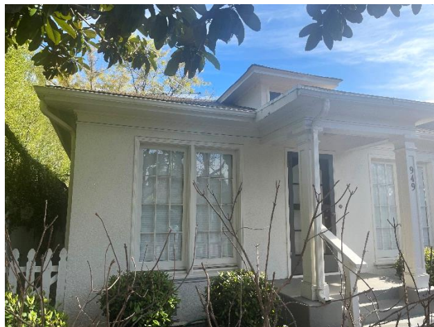
Figure 2: North half of southwest facade.
