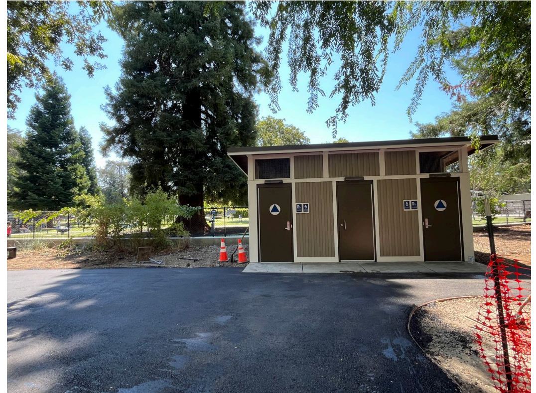
Rinconada Restrooms - OPEN
