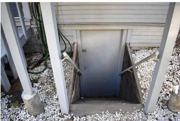
Figure 8: Steps to basement from rear south façade.
