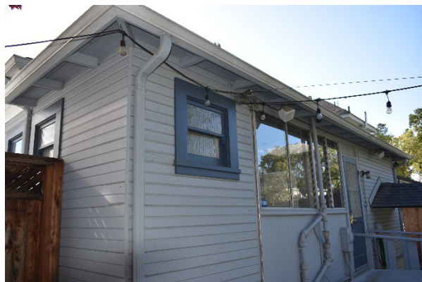
Figure 9: Oblique view of the rear north façade, looking west.
