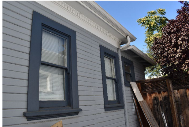
Figure 12: Detail view fenestration at northern section on the east façade, looking north.
