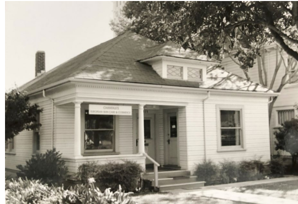
Figure 37. 411 Kipling Street, 1999. Source: B. Vahey, Palo Alto Historical Association.
