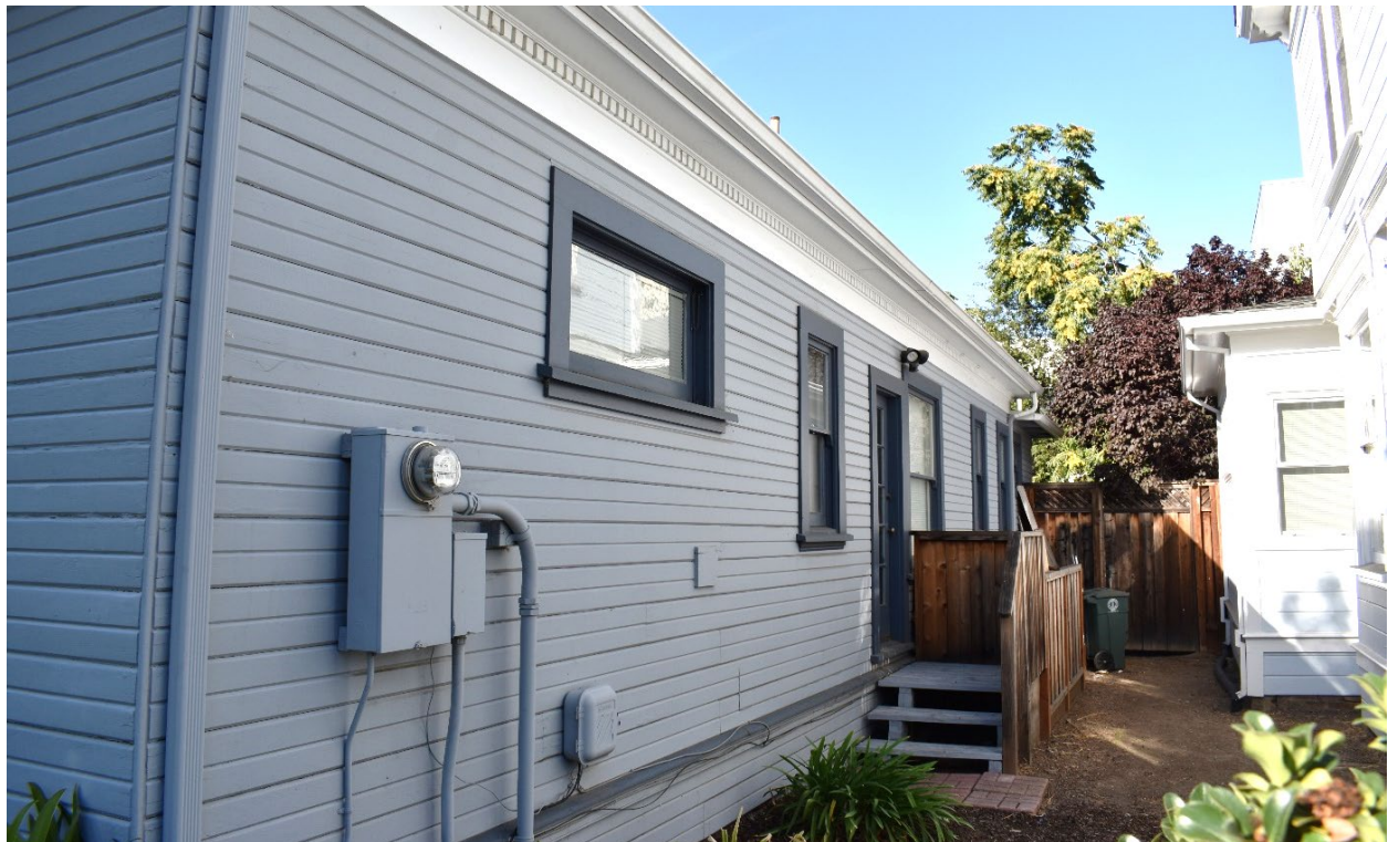
Figure 10: Oblique view of east façade, looking north.
