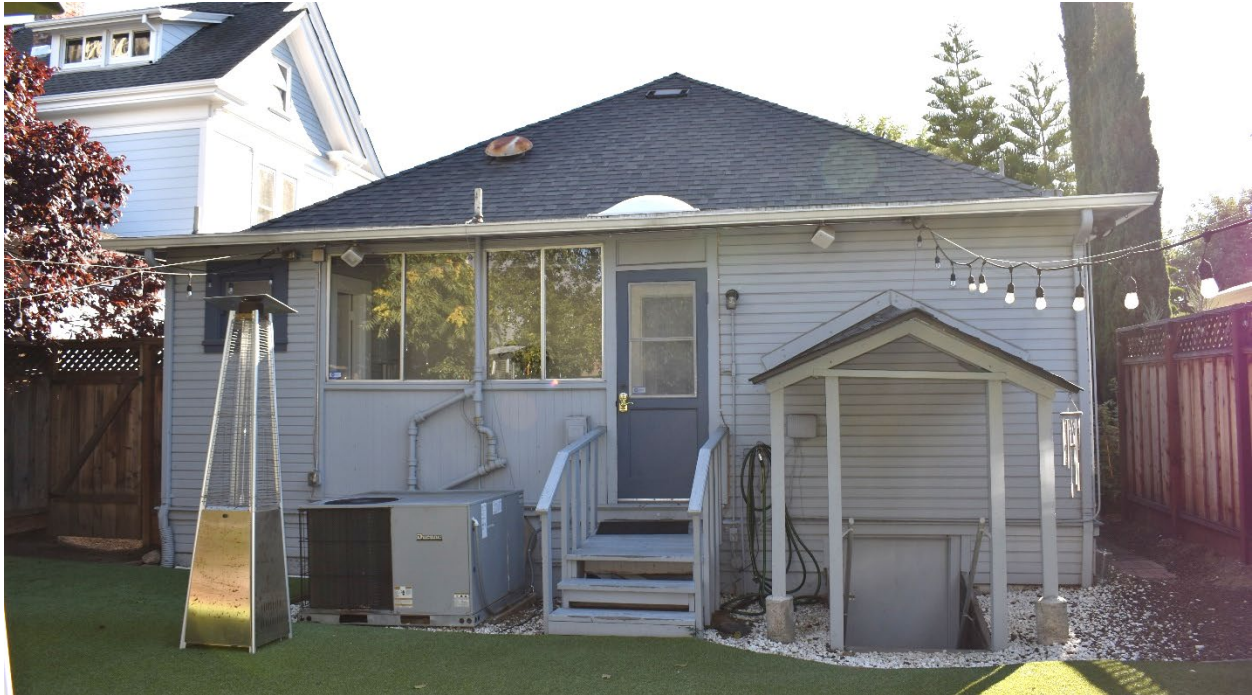
Figure 7: Rear north facade of 411 Kipling Street, looking southwest.
