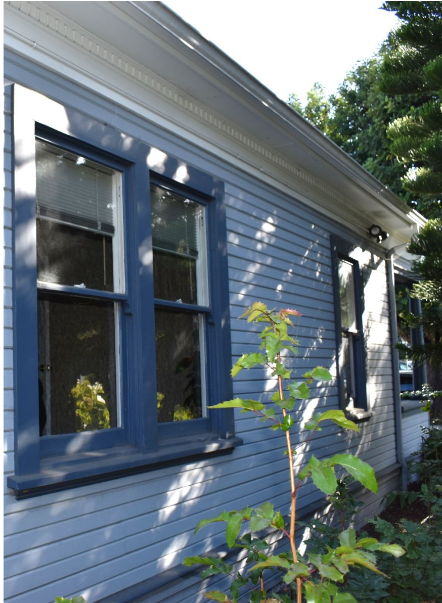
Figure 6: Oblique view of the west façade, looking south.
