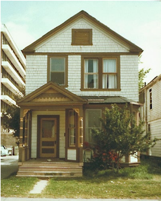
Figure 20. 617 High Street (1897), builder George W. Mosher. Source: Palo Alto Stanford Heritage, c.1986
