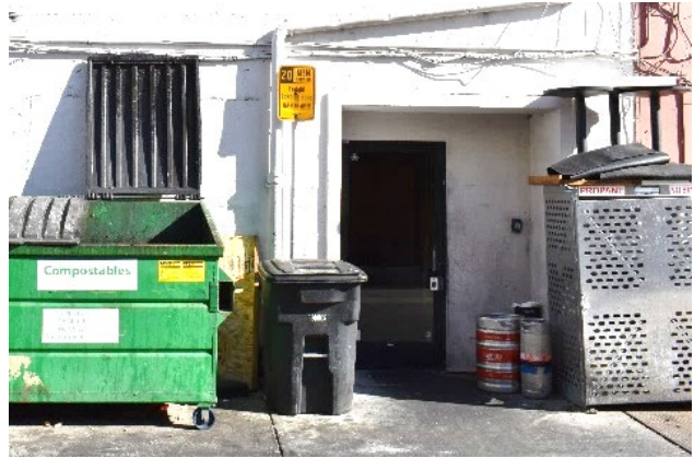
Figure 10. Entryway of the rear façade, facing southeast.
