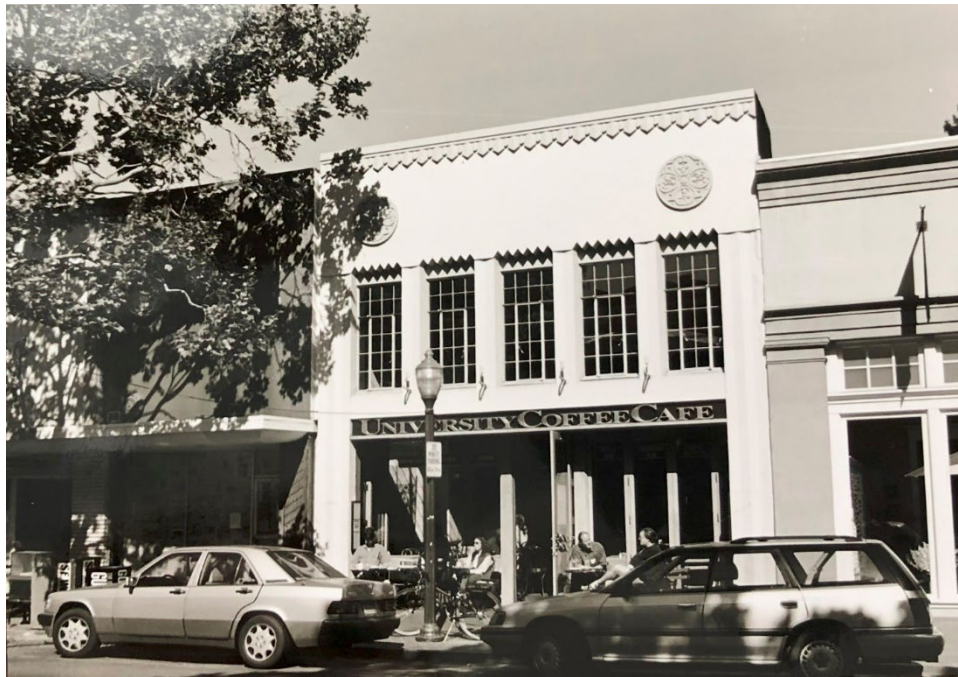
Figure 30. Subject building, 1999. Source: Palo Alto Historical Association.
