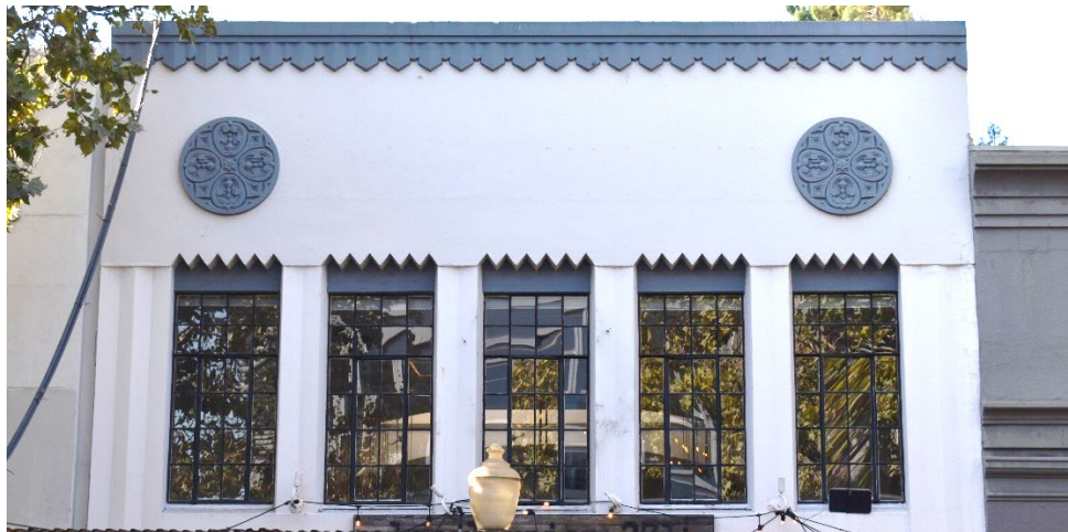
Figure 6: Casement windows, medallions, and cornice at the upper floor level of the primary façade.
