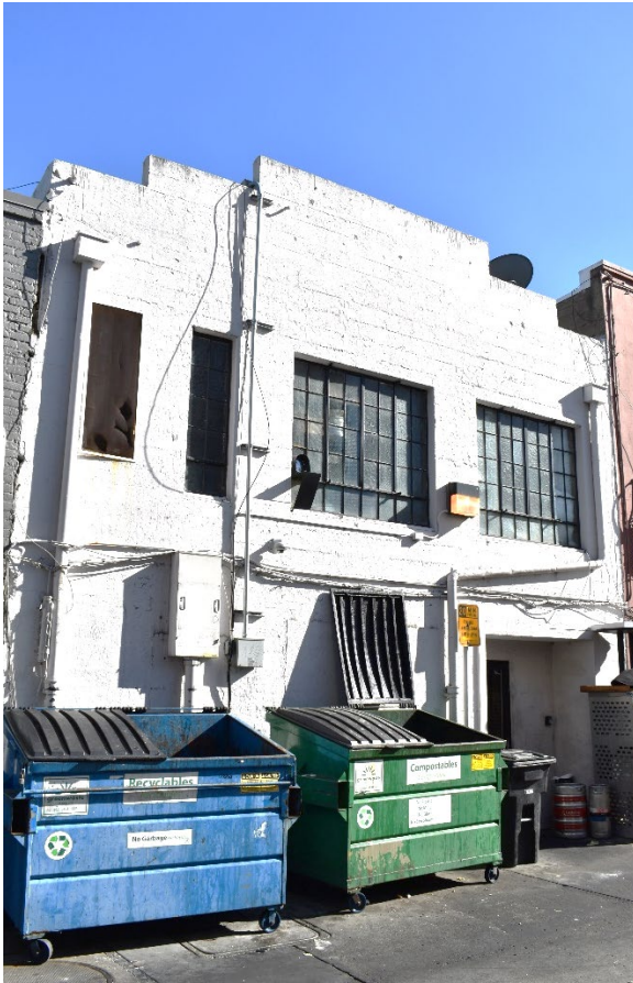
Figure 9. Oblique view of the rear façade, looking south.
