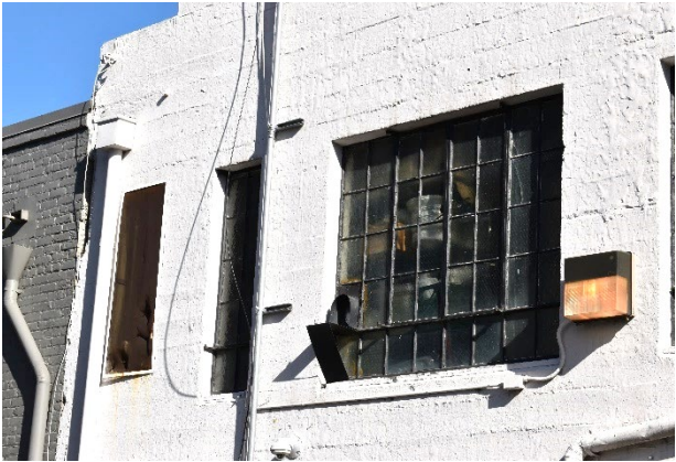
Figure 12: Detail view of casement windows at the upper floor of the rear façade, facing east.
