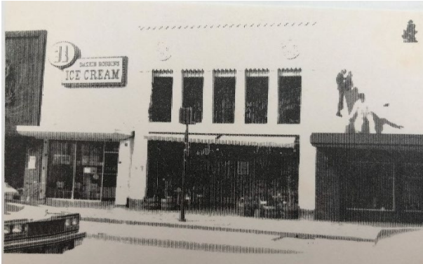
Figure 28: Historic Resources Inventory photograph of 271 University Avenue, 1978. Source: Palo Alto Historical Association.
