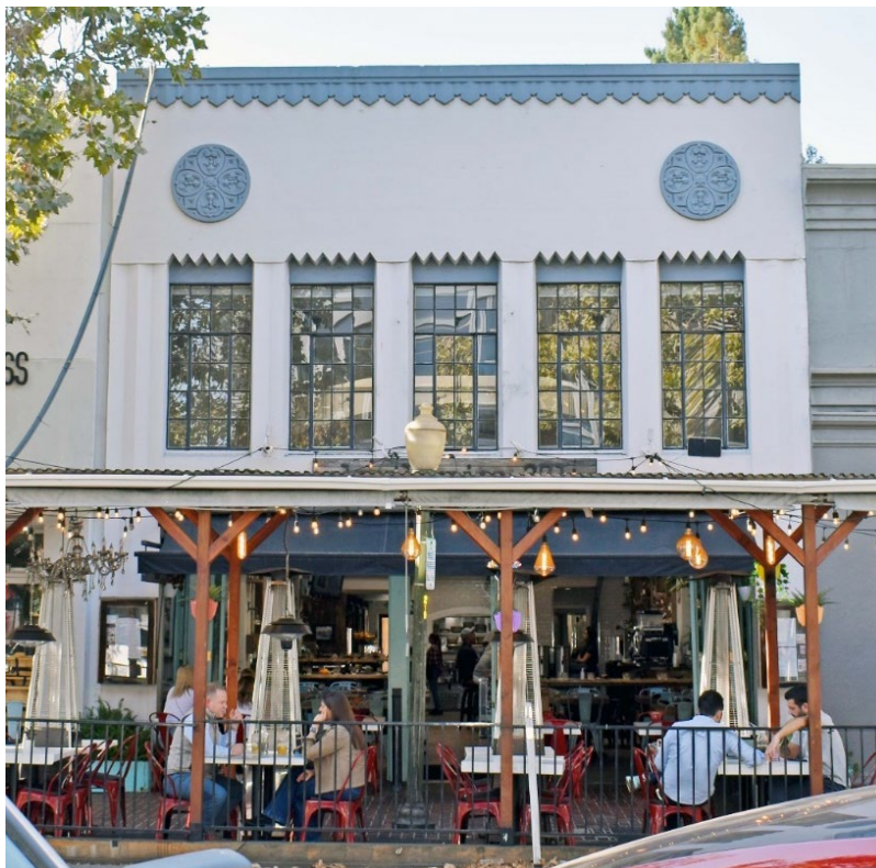
Figure 3: Primary façade of 271 University Avenue.
