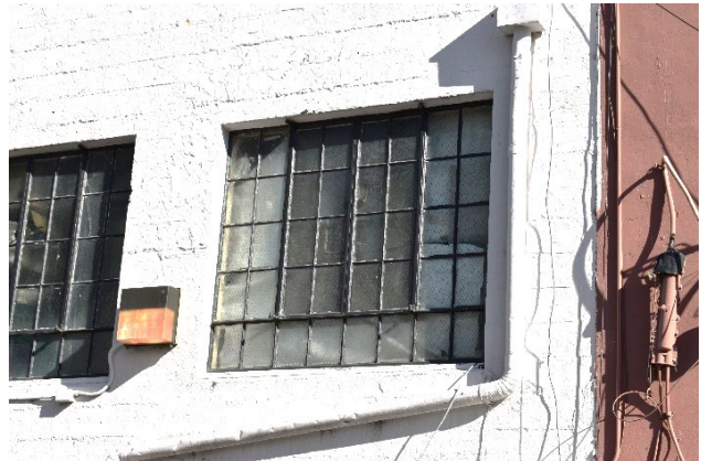
Figure 11. Detail view of casement windows at the upper floor of the rear façade, facing east.
