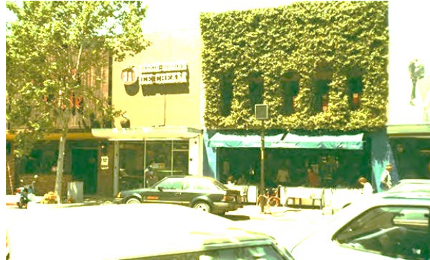
Figure 29. Subject building, 1985. Source: Palo Alto Historical Association.
