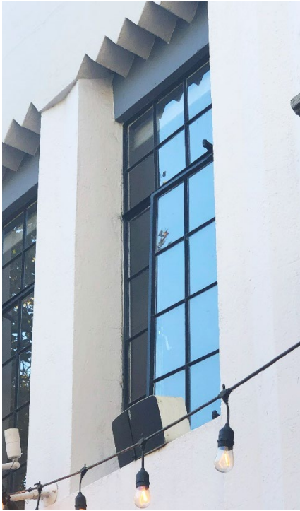
Figure 7: Detail view of casement windows at the second-floor level.
