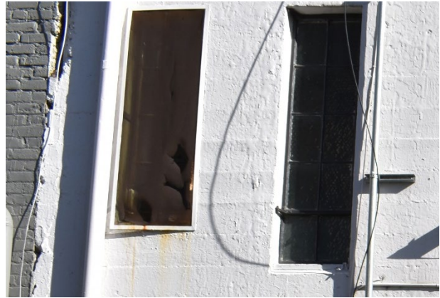
Figure 13: Detail view of smaller casement windows at the upper floor of the rear façade, facing east.
