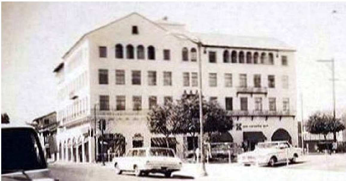
Figure 10. Context view of the south and east facades at the corner of Ramona Street and Hamilton Avenue, c. early 1960s. Source: Palo Alto Historical Association.
