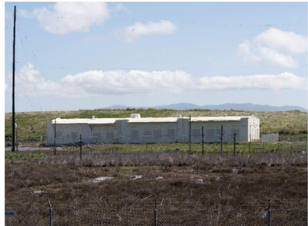
Figure 2: 2023 Reconnaissance Survey photograph.
