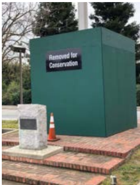
Plywood box enclosing Memorial Flagpole
