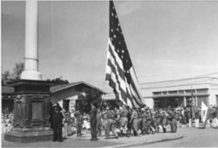
University Ave Underpass Opening Celebration, 1941
