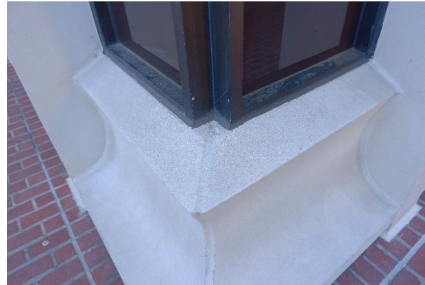
Figure 21. Curved concrete base and fillet joint corner at windows.
