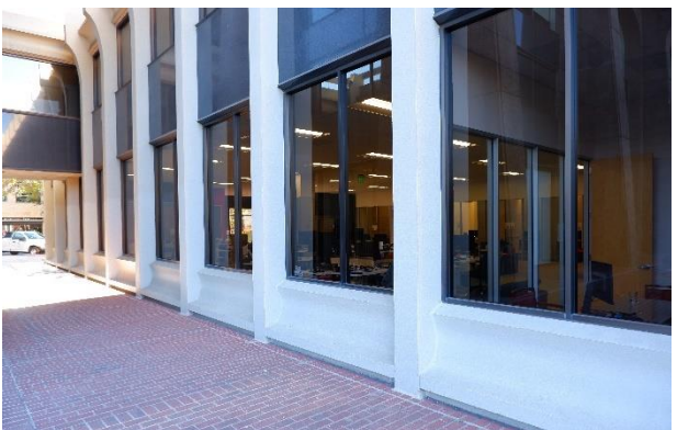
Figure 30. Pedestrian bridge at second bay of the south façade.
