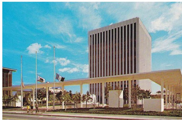
Figure 56. Postcard of Palo Alto City Hall by Edward Durrell Stone, completed in 1967. Source: Flickr.com.
