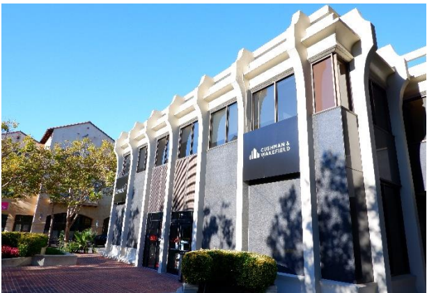
Figure 26. East façade of the South Wing.
