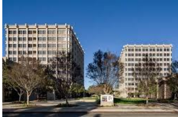
Figure 58. Palo Alto Square, 3000 El Camino Real, designed by Albert Hoover in 1972. Source: Hudson Pacific Properties.
