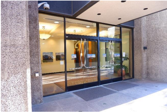
Figure 11. South lobby entrance, below the enclosed pedestrian bridge, looking northeast.
