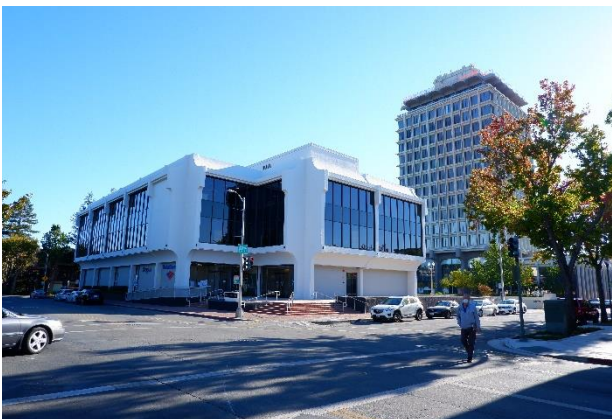
Figure 48. Commercial building at 530 Lytton Avenue, looking northeast from intersection with Cowper Street.
