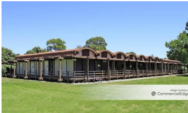
Figure 61. Sunnyvale Office Center at 505 West Olive Avenue, Sunnyvale, designed by Tallie Maule. Source: CommercialEdge.
