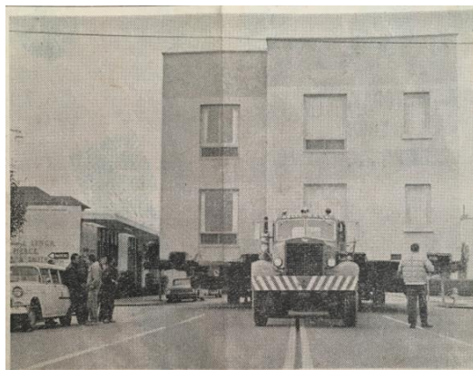
Figure 63. Former office of Hare, Brewer & Kelley, originally located at 525 University Avenue, being relocated to make room for Palo Alto Office Center. Source: "Big moving job," Palo Alto Times , December 31, 1963.
