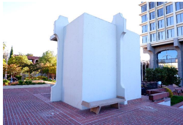
Figure 41. South side of the elevator structure, looking northeast.
