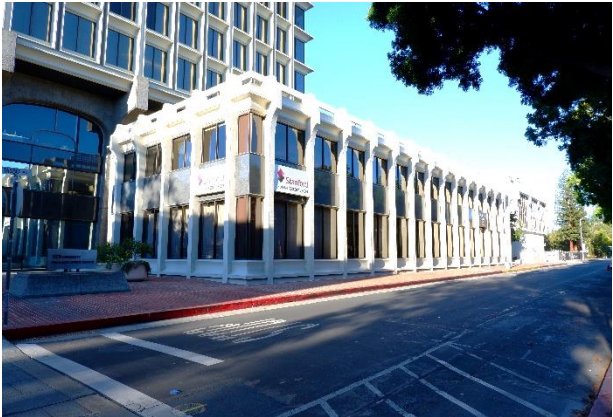
Figure 20. East and north facades of the North Wing, looking southeast.
