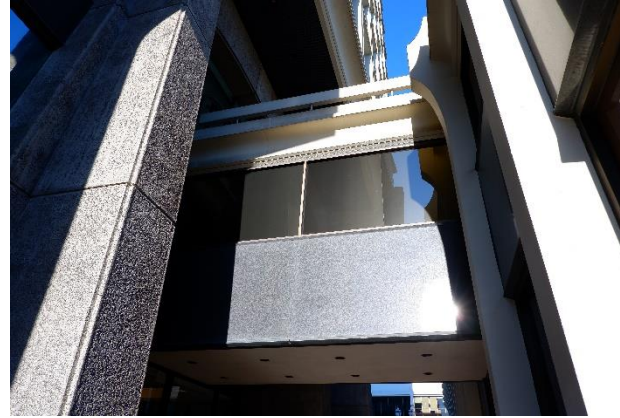
Figure 25. Enclosed pedestrian bridge connecting Office Tower (left) and North Wing (right) at second story.
