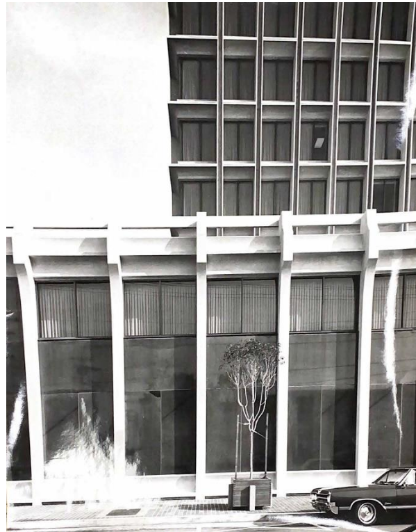
Figure 72. South façade of the South Wing, featuring black granite panels at the first floor due to interior banking function, circa 1966. Source: University of California, Berkeley, Environmental Design Archives.
