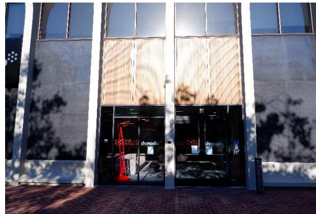
Figure 27. Corrugated metal panels over the doors.
