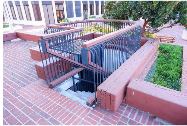
Figure 39. Upper level staircase to the underground parking garage.
