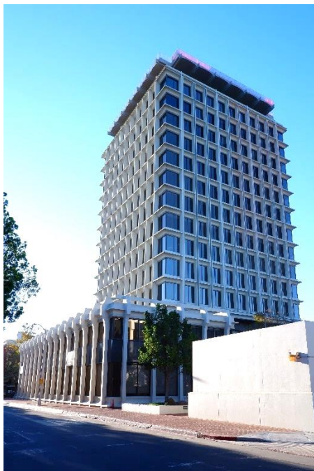
Figure 15. North (left) and west (right) facades of the office tower shaft, looking southeast down Tasso Street.
