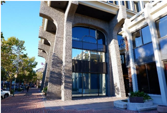
Figure 5. Bush-hammered concrete columns at base of office tower, looking southwest.
