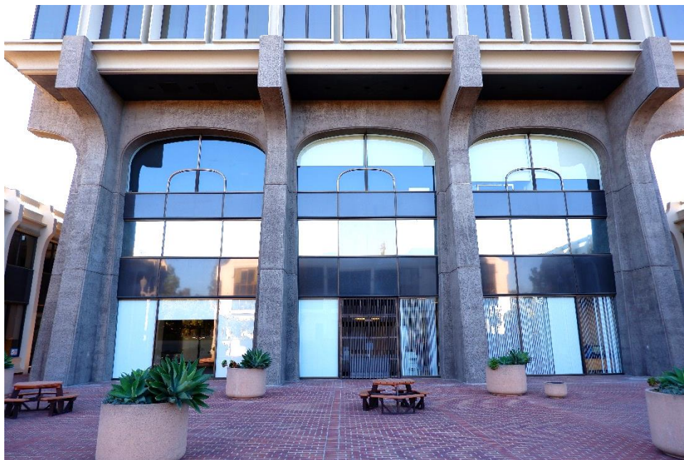
Figure 8. Base at the west façade of the office tower, looking east.
