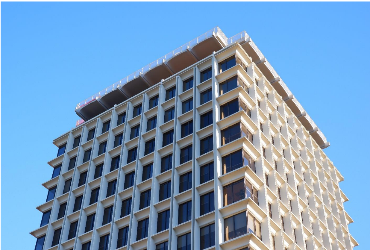
Figure 18. Cantilevered penthouse roof at the 15 th story of the office tower.
