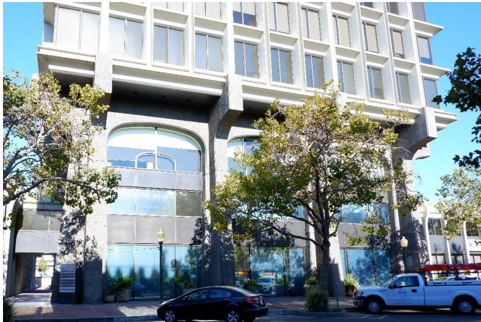
Figure 7. Base at the east façade of the office tower, looking northwest.
