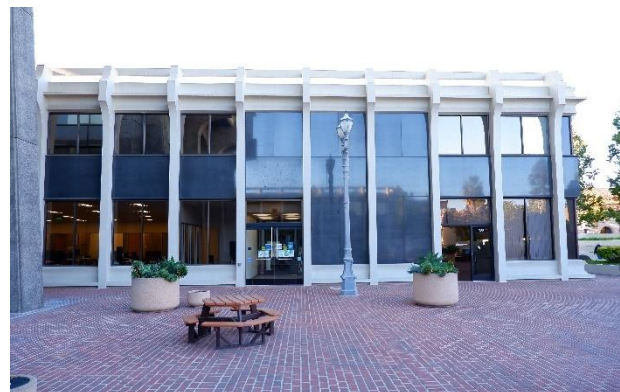
Figure 31. Doorways at the tenth and thirteenth bays of the south façade.
