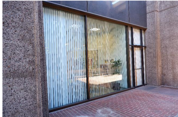
Figure 10. Non-original exit door at south façade.
