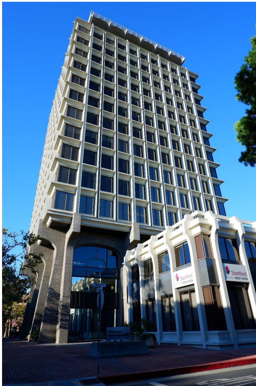
Figure 4. Main office tower and connected north wing, looking southeast.
