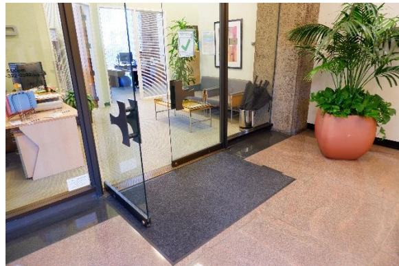
Figure 14. Ground floor office tenant space, accessed from the lobby, with shaped bronze anodize aluminum door handles.
