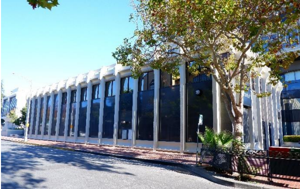
Figure 28. South façade of the South Wing, looking northwest.
