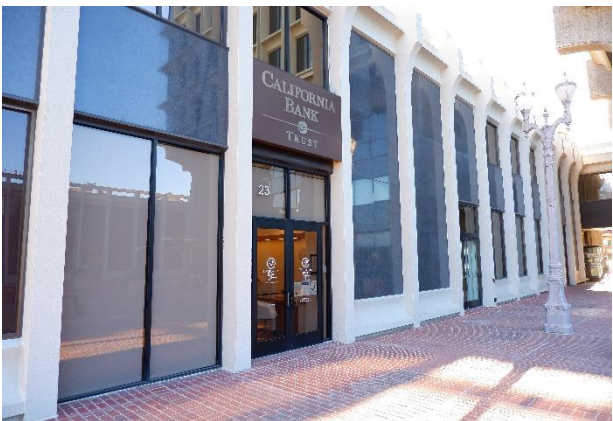
Figure 22. Doorways at south façade of the North Wing, looking northeast.
