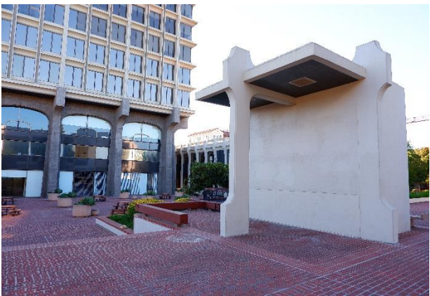
Figure 40. North side of the elevator structure, looking southeast.
