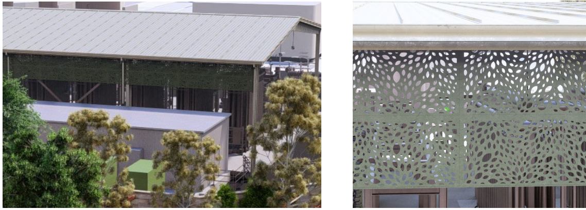
Figure 1. Architectural aluminum panel for increased screening and to prevent light dispersion
