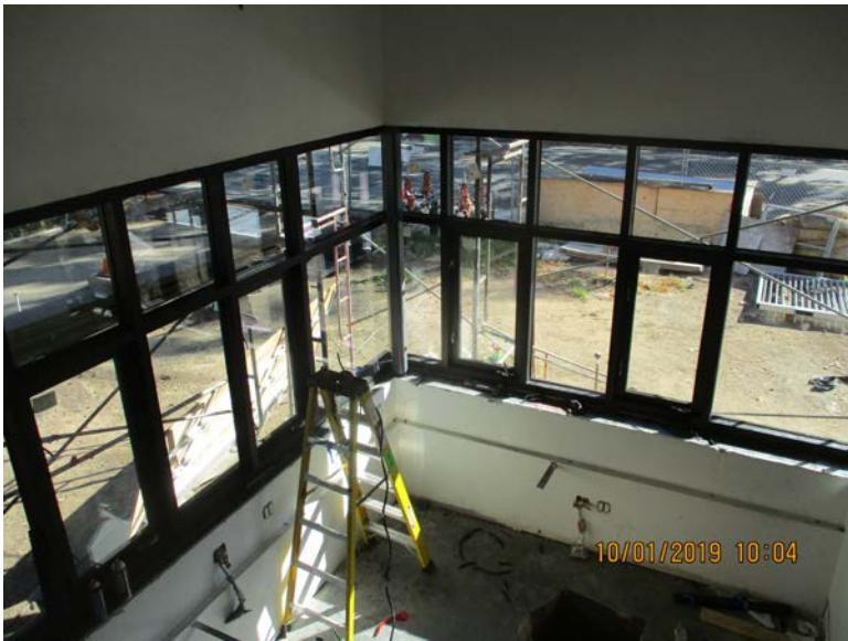
Watch room glass installed
