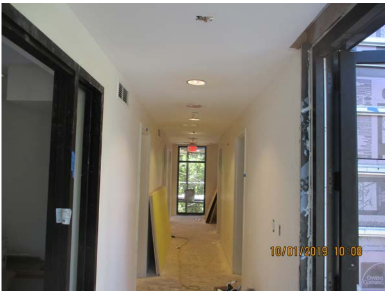
Interior finishes in progress
