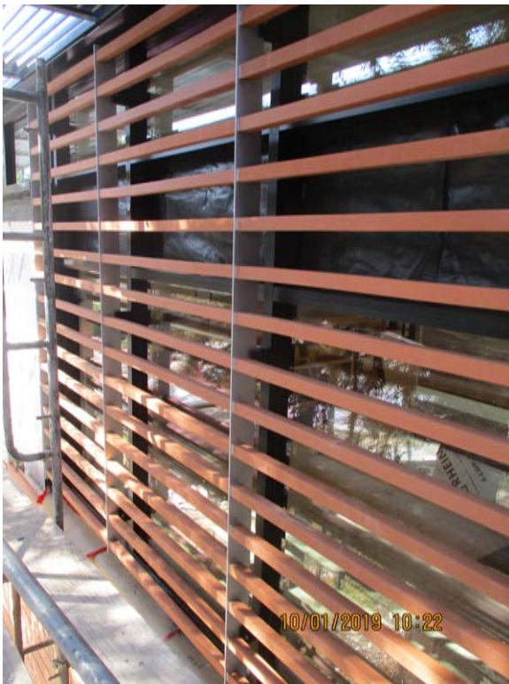
Terraclad baguette installation at dining room
