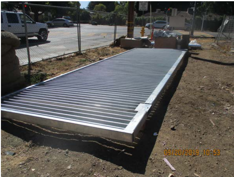
Delivery of rolling gate for back of house entrance
