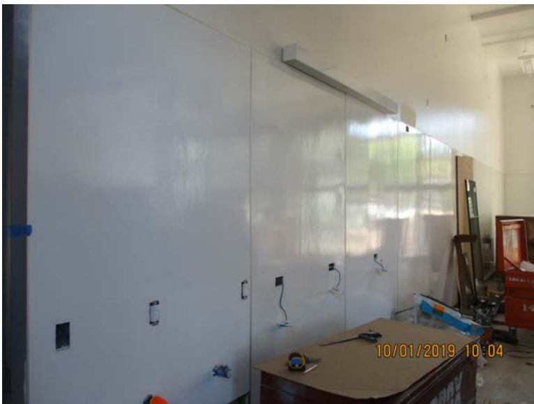
FRP installation in apparatus bay
