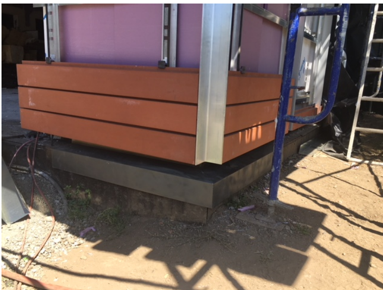
Outside corner mockup for terra cotta.
