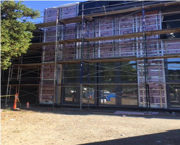
Rigid foam insulation and channels installed for terra cotta.
