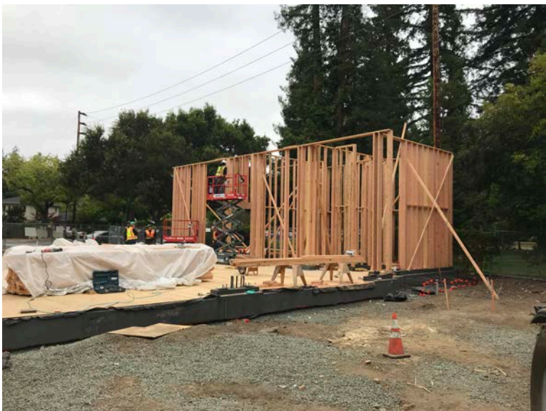
Structural framing continuing on west side.
