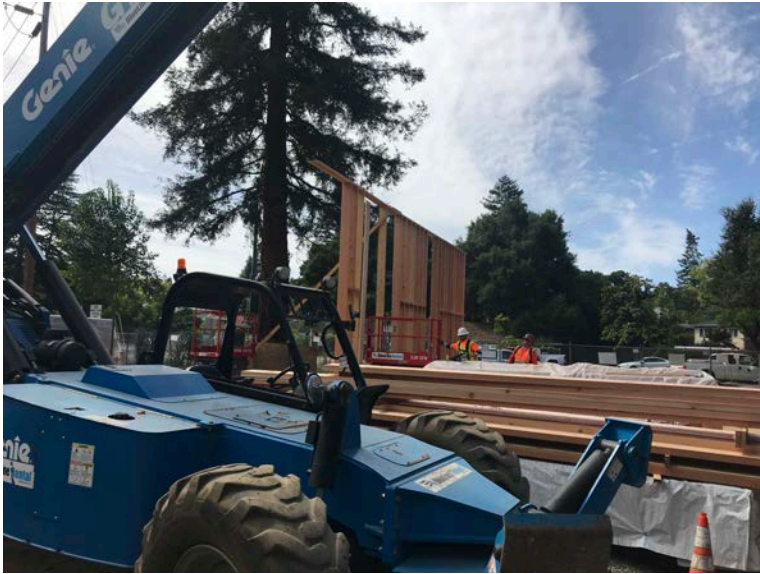
Wood framing started on east side.
