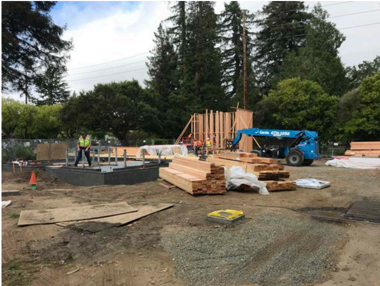
Structural wood framing started for first story of the new structure.
