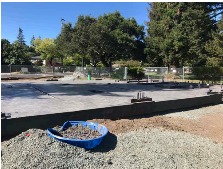
Mat slab forms stripped.
