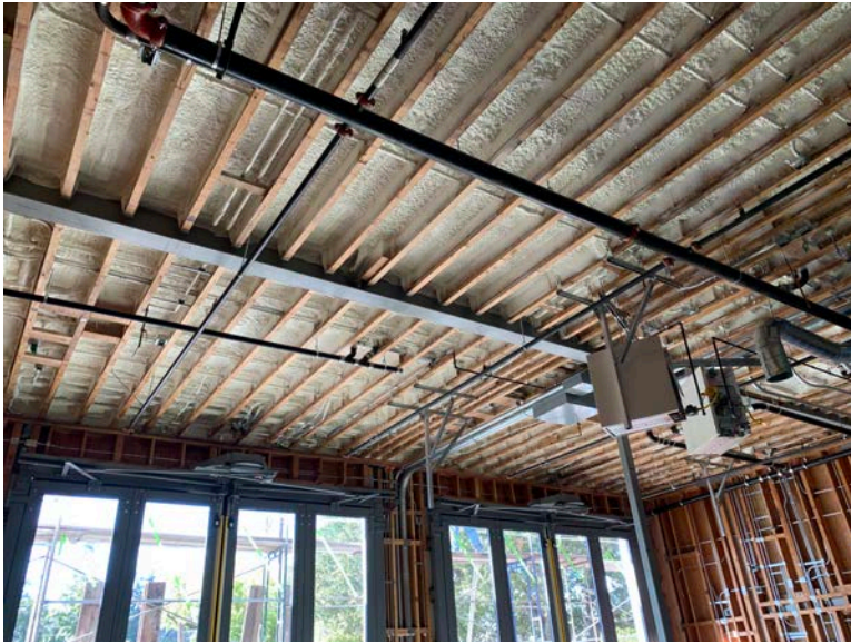
Spray insulation in apparatus bay.
