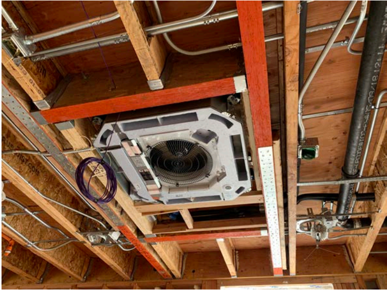
Exhaust fan in exercise room.
