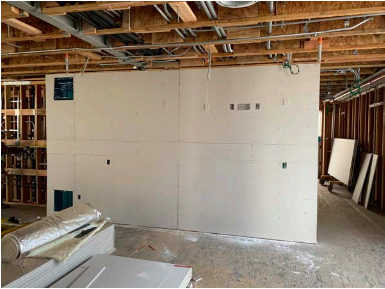
Drywall install started on 2 nd Floor.
