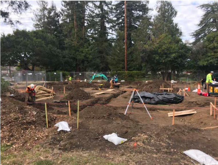
Underground Utilities excavation.
