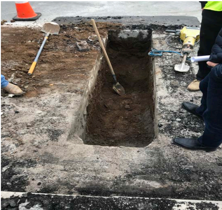
Potholing of Newell Rd for sewer tie-in.
