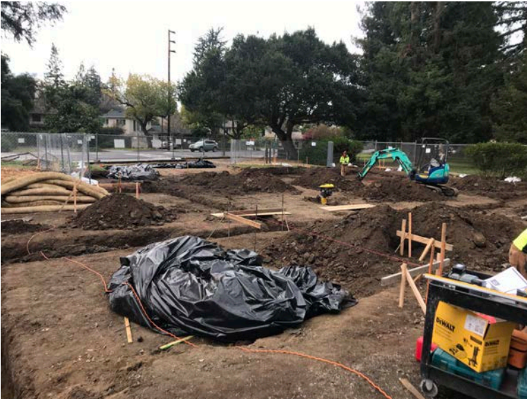
Underslab utility excavation.
