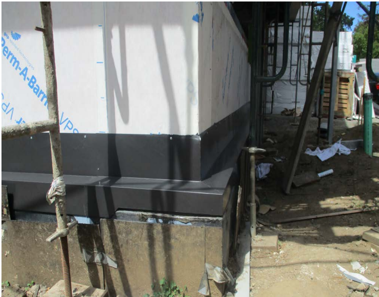
Ongoing aluminum base flashing installation.
