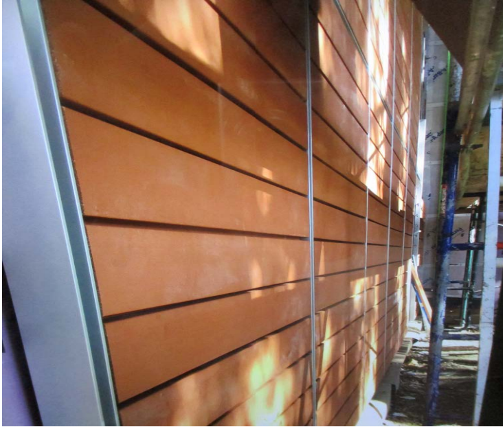
Terra Cotta wall panel installation.
