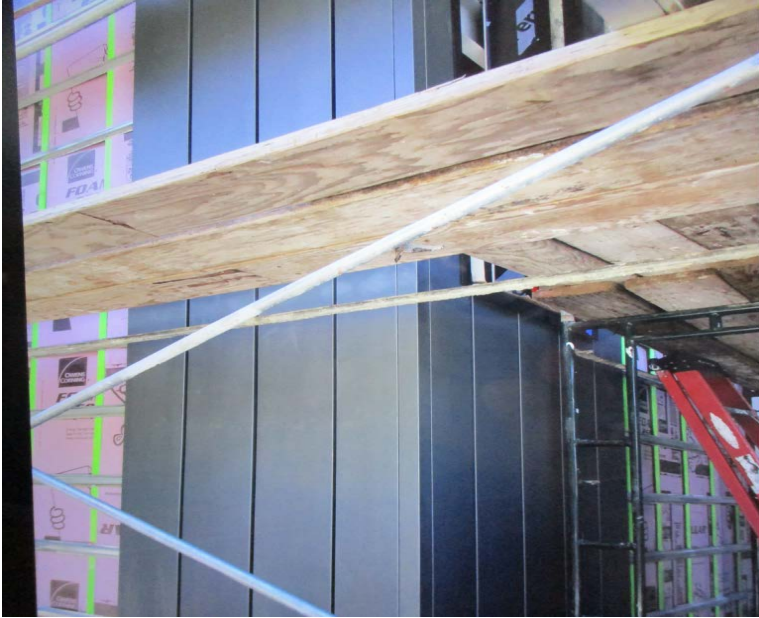
Zinc Panel Mockup.
