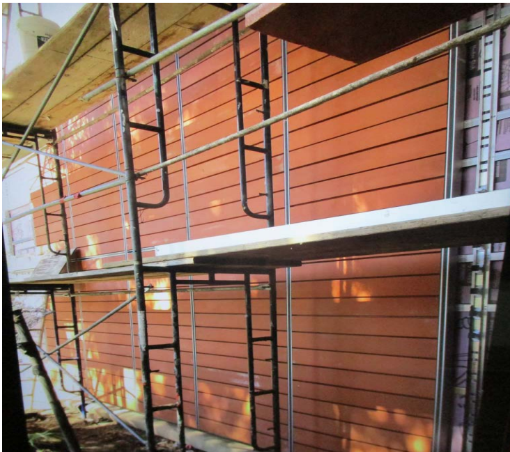
East Elevation Terra Cotta Wall panel installation continued.
