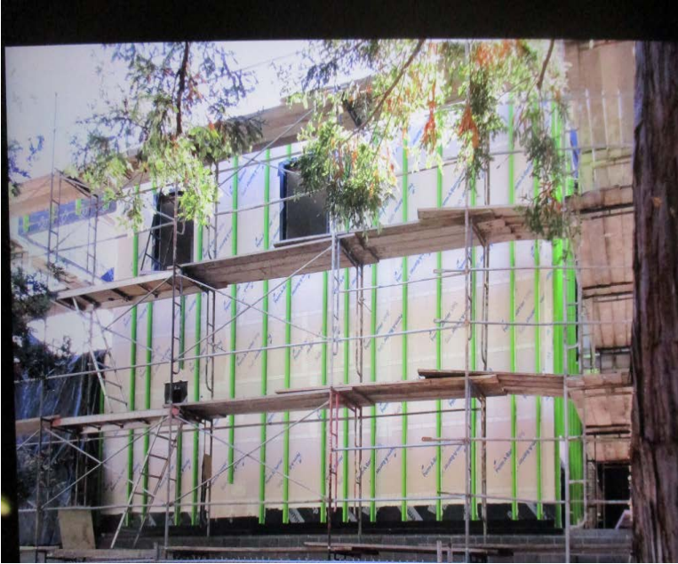
Green Girt installation at west elevation.
