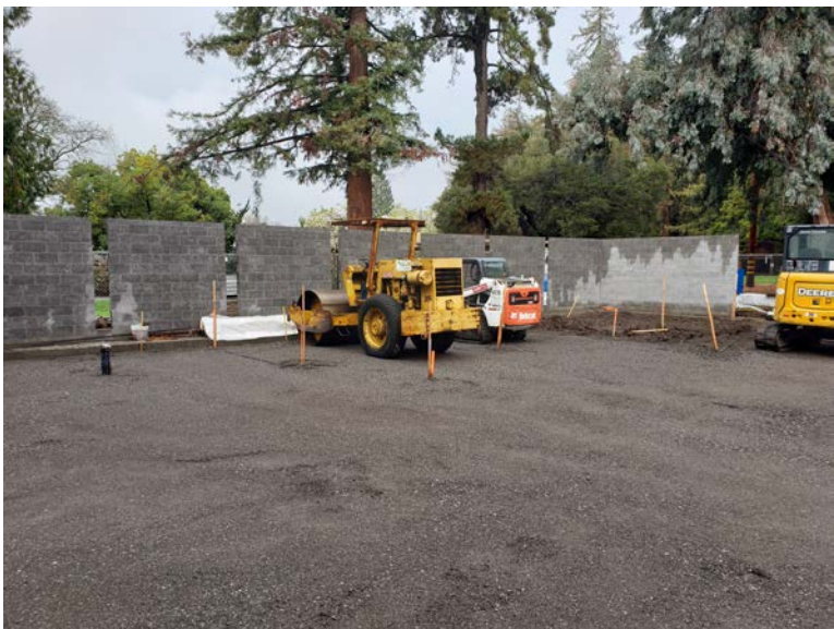
Hard grade of back parking lot.
