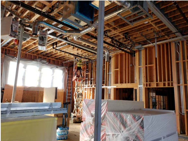
M-E-P Rough in in Apparatus Bay. Drywall delivery.
