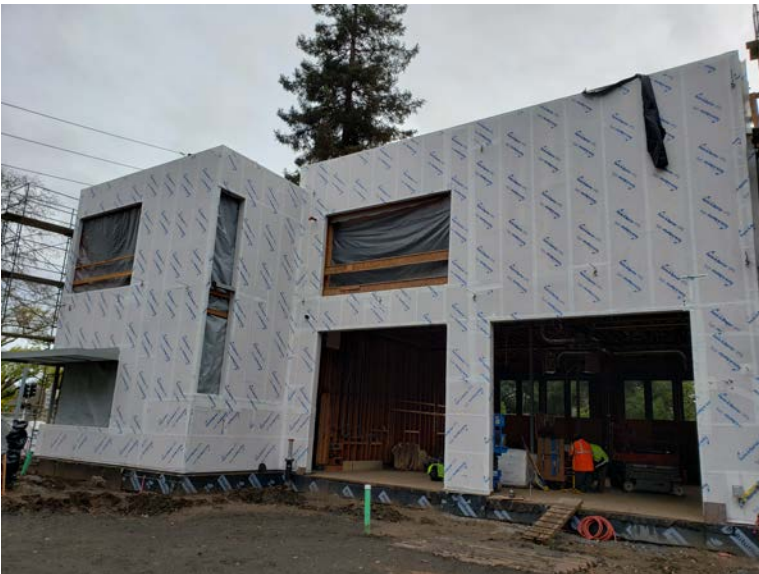
Waterproofing on North side of structure.
