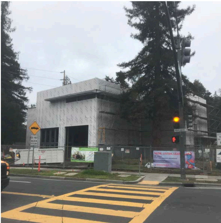
Fire station from Embarcadero.
