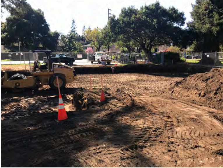
Excavation and grading for the future building pad.
