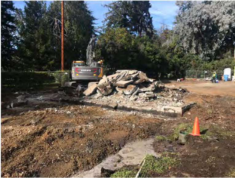
Demolition of site asphalt and existing foundation.
