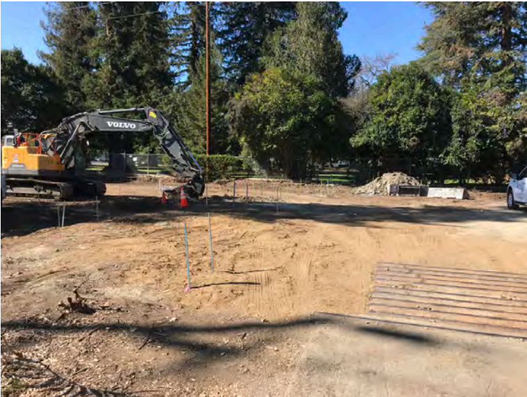
Survey staking for underground utilities.
