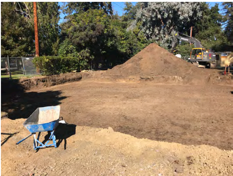
Building pad compaction complete.
