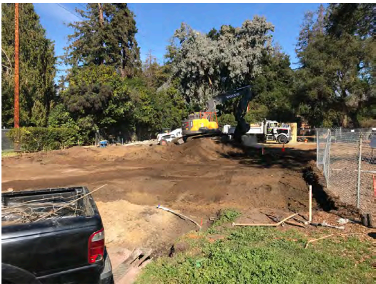
Site grading ongoing following completion of demolition.
