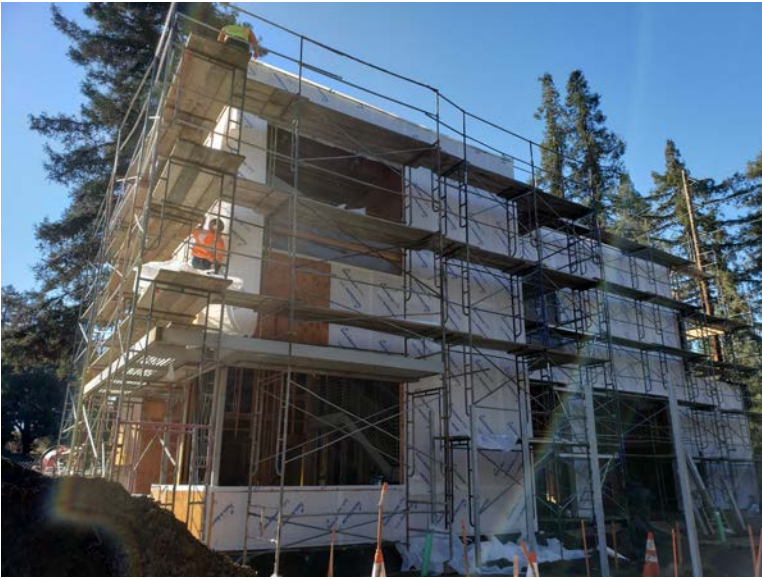
Exterior waterproofing install on north side.
