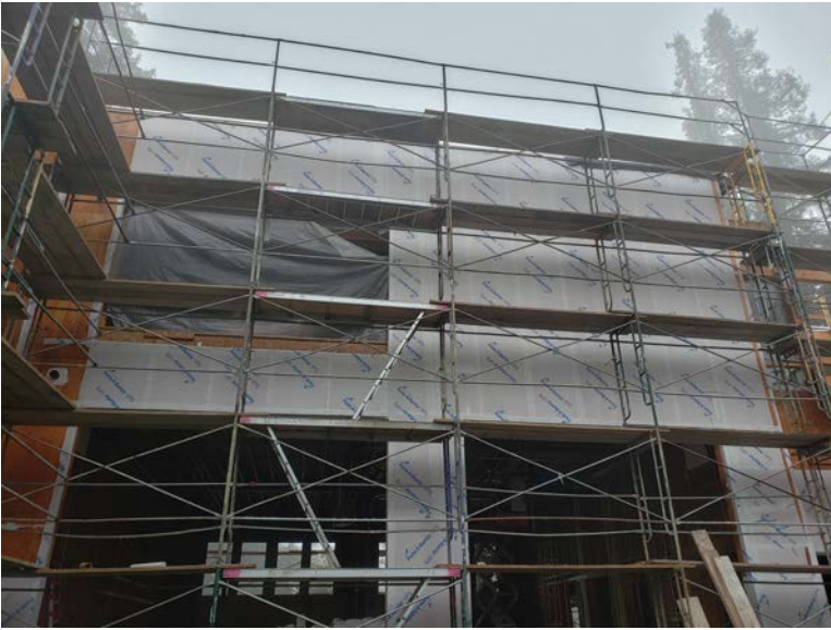
Exterior waterproofing install with scaffolding.
