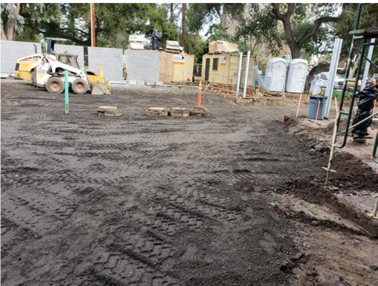
Grading of back parking lot.
