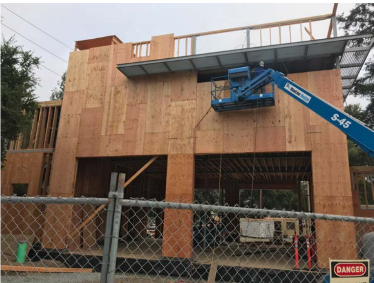
Exterior framing and sheathing of Embarcadero side of the building.
