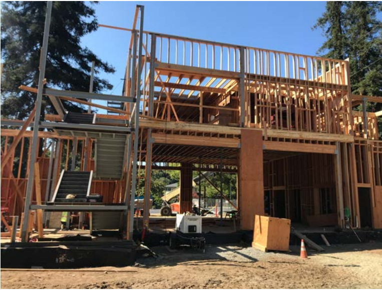
Continued structural framing including roof parapet.
