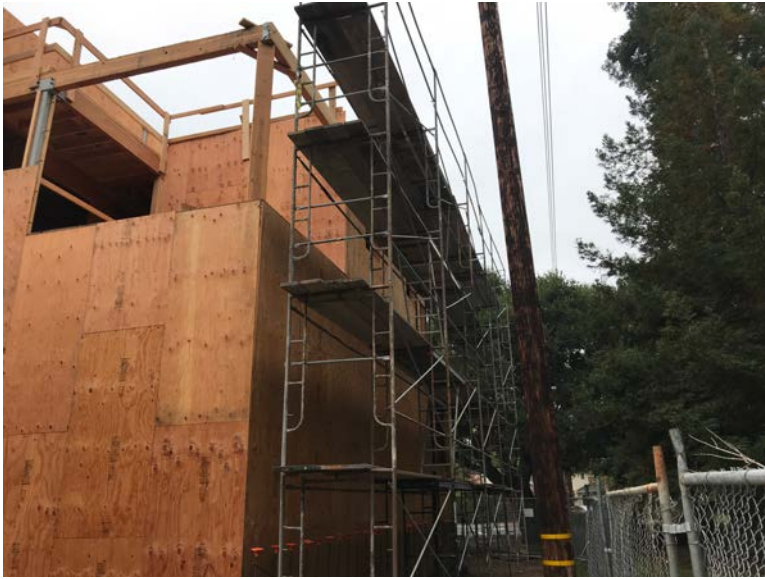
Scaffolding installed onsite, park side.
