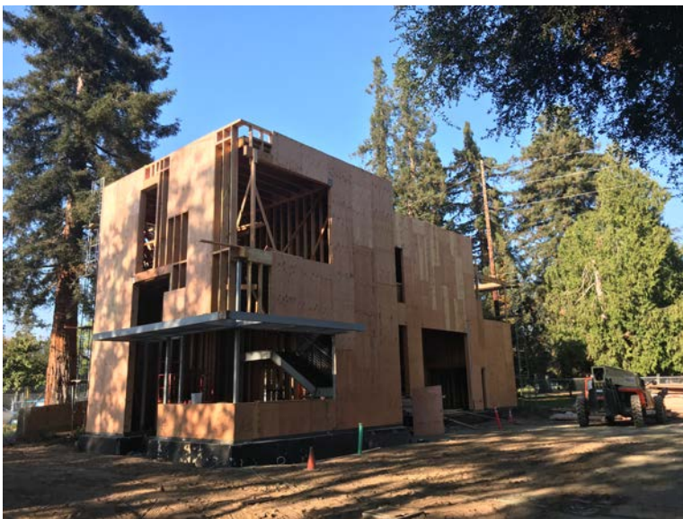
Exterior Sheathing on North side.
