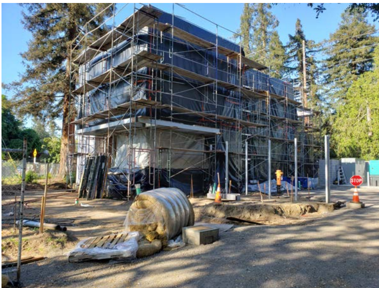
Exterior waterproofing protection from UV exposure.
