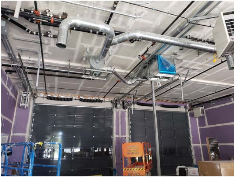
Drywall mud/tape activities at Apparatus Bay.
