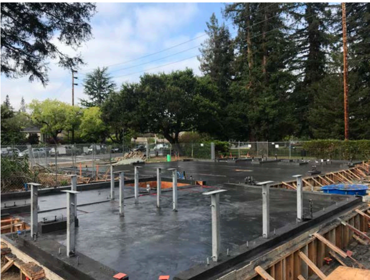
Mat Slab curing the day following the pour.
