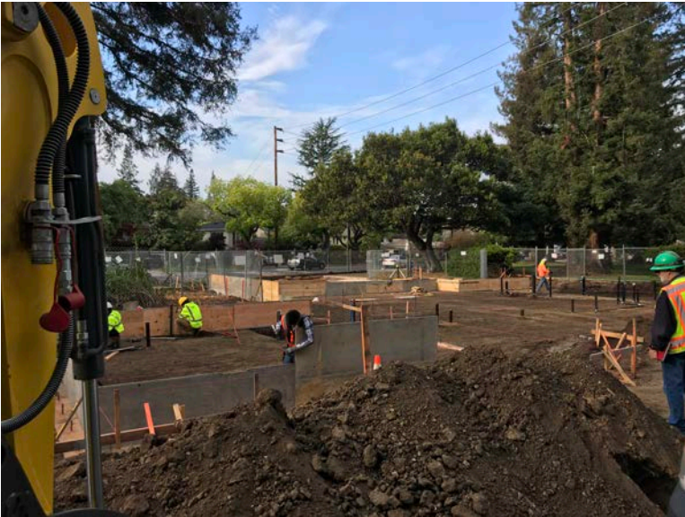
Mat Slab Form Work Started.
