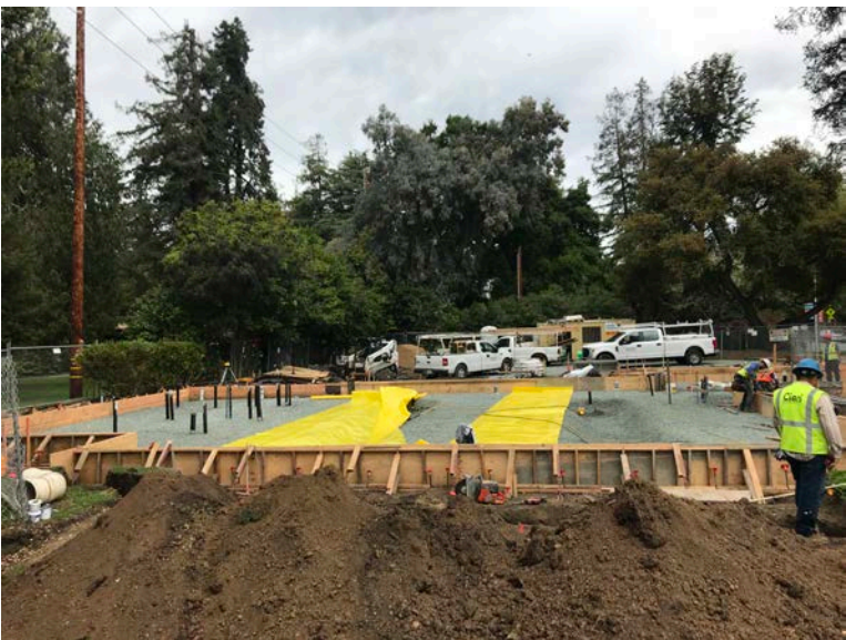
Mat Slab base rock installed, vapor barrier started.
