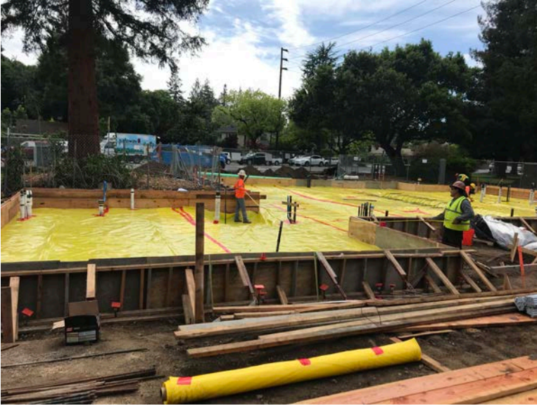
Mat Slab Vapor Barrier Installed.
