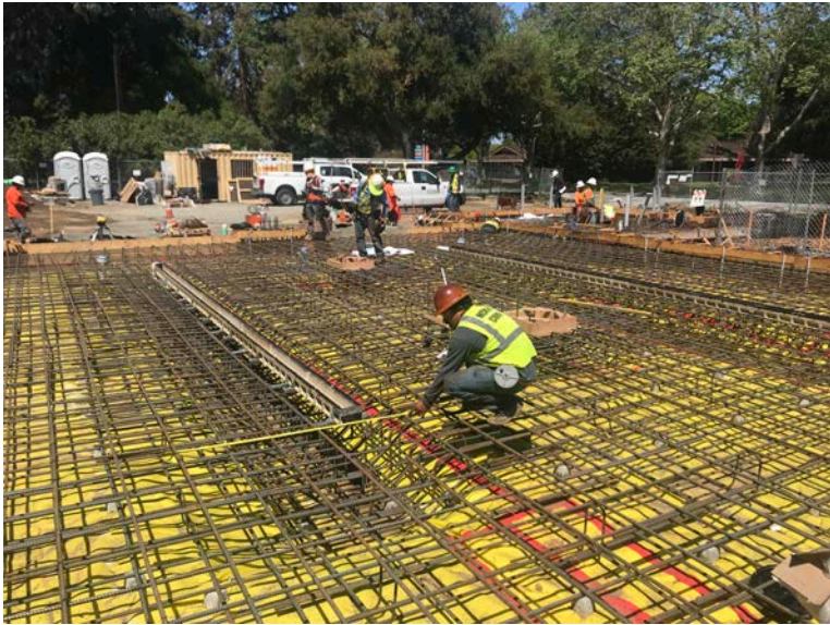
Mat Slab Rebar Substantially complete.
