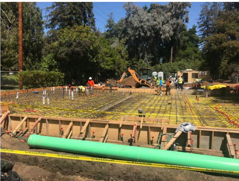
Mat Slab rebar being installed.
