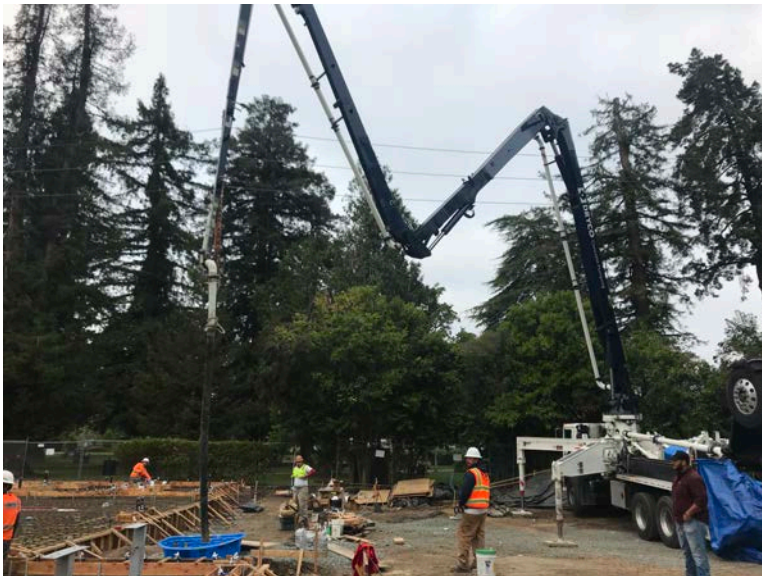
Mat Slab Concrete Pump Truck.
