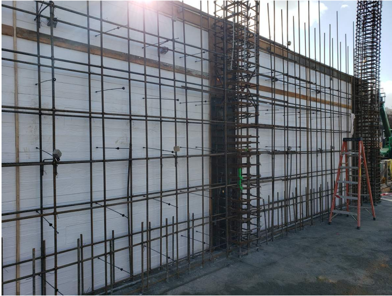
“Board form” cast-in-place wall being formed.
