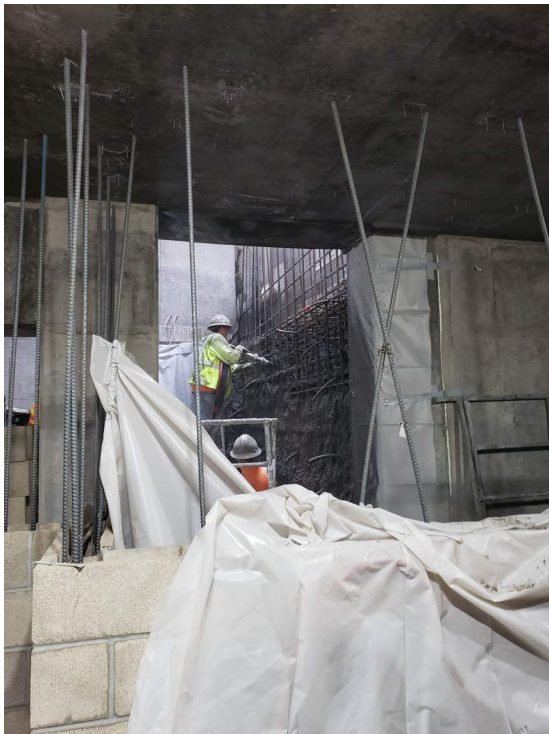
Shotcrete activities commencing in the B2 level.
