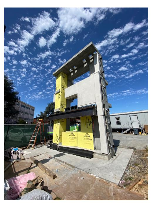
Drywall, miscellaneous metal, and precast concrete panels installed on the mock-up that is adjacent to jobsite.
