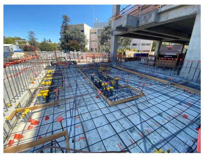
Structural foam, rebar, conduits, and formwork in place in the Utility Yard.
