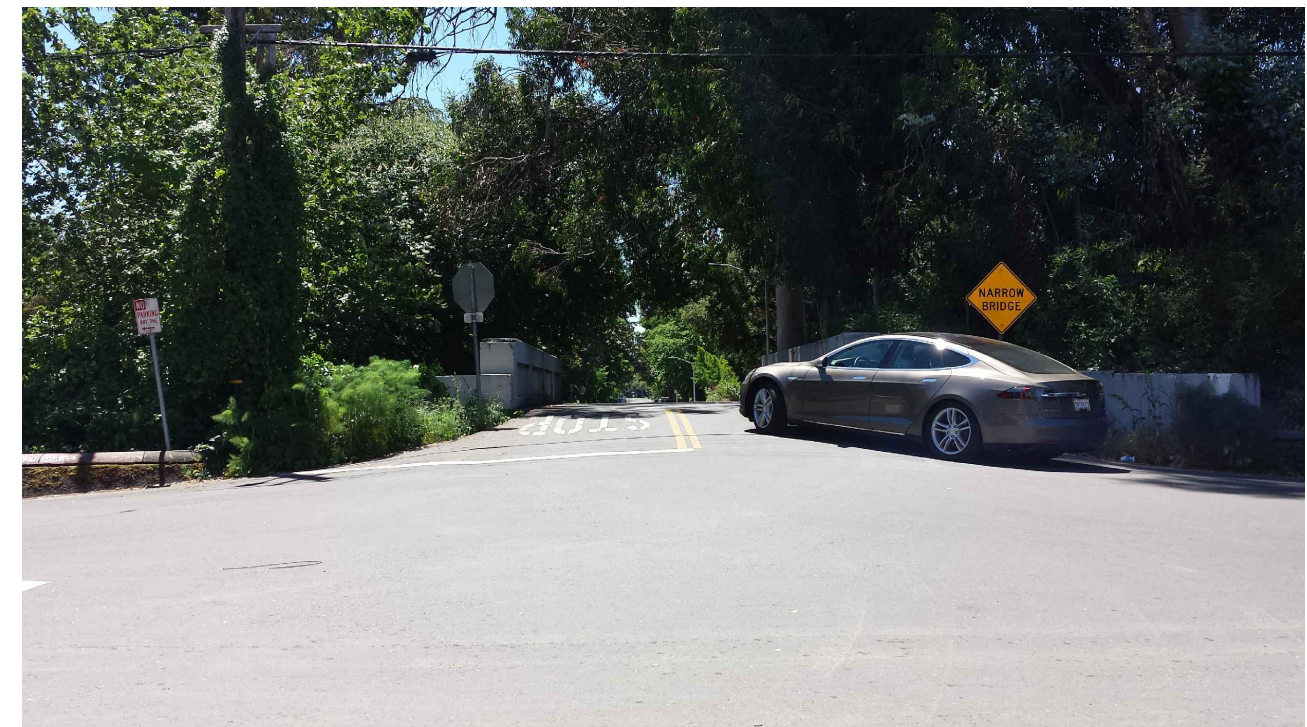
IMAGE 4: NEWELL BRIDGE VIEW FROM EAST PALO ALTO
