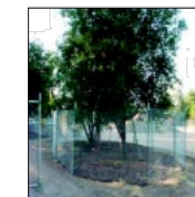
IMAGE 2.15-1 Tree Protection Fence at the Dripline
