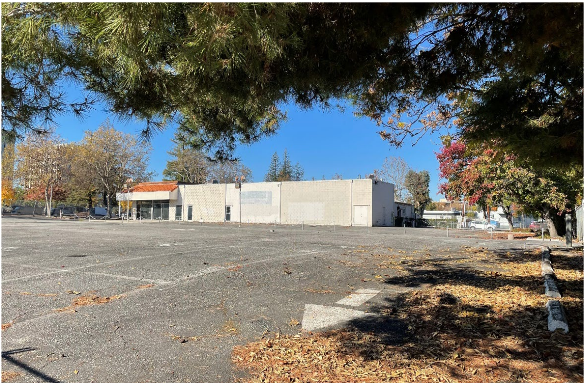
Photograph 4. View of the existing structure from the northeast corner of the project site looking southwest.
