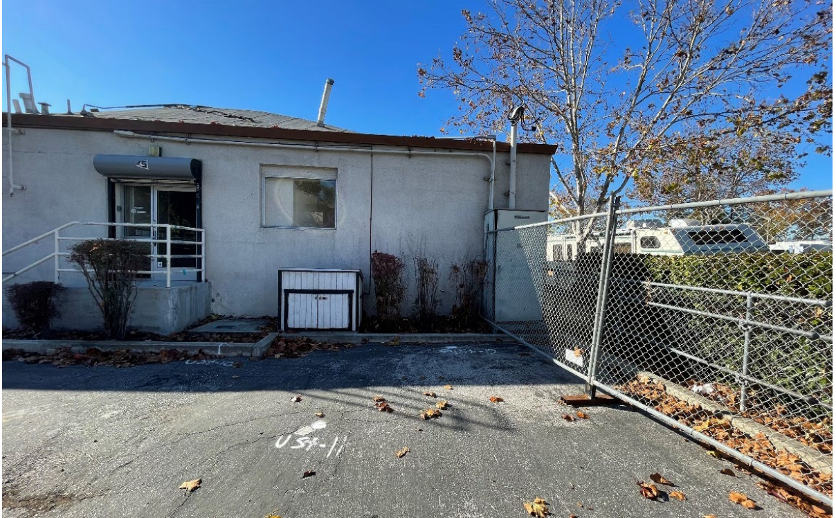
Photograph 3. View of the existing structure from the northern portion of the project site looking south.
