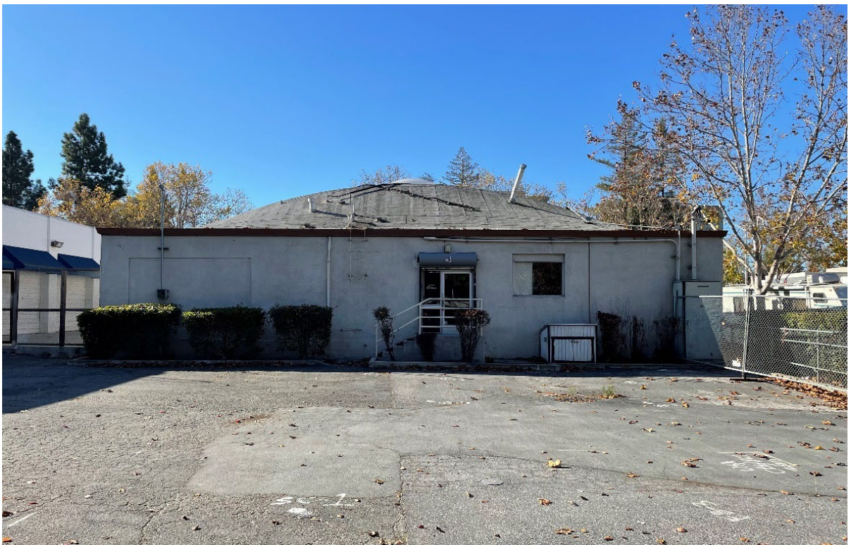
Photograph 2. View of the existing structure from the northern portion of the project site looking south.
