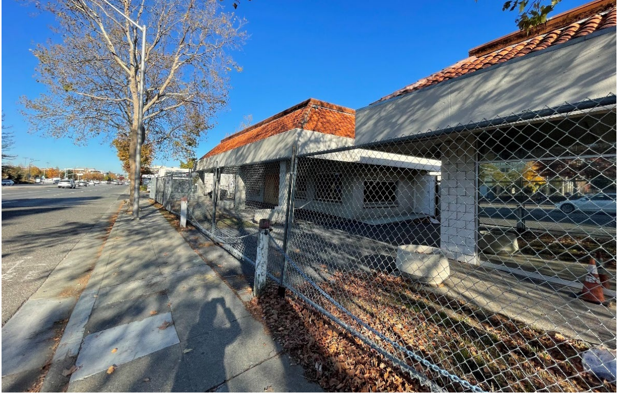
Photograph 1. View of the existing structures from El Camino Real looking north.
