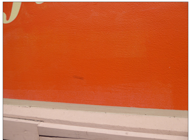
Detail of water staining and scuff marks.
