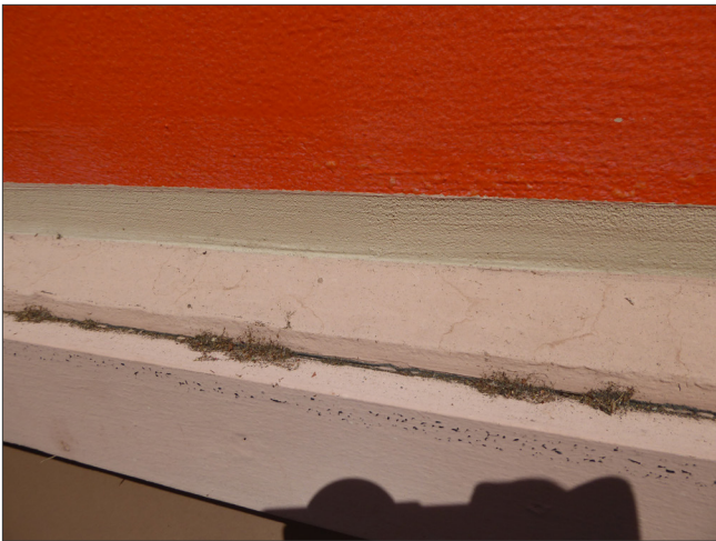
Detail of biogrowth at sill.
