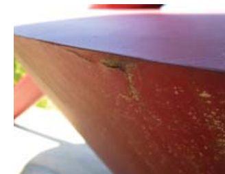
Detail of paint peeling and corrosion at edge of circular piece.
