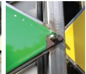
Detail of corrosion at panel fastener location.
