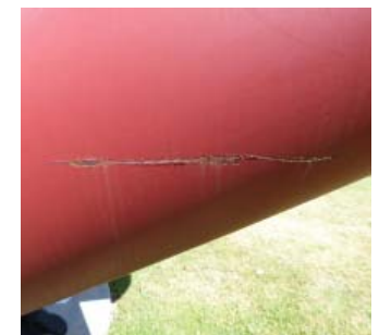
Detail of gouge at front of tube. Note peeling paint and corrosion.
