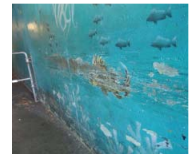
Detail of paint loss/ abrasion at tunnel walls.
