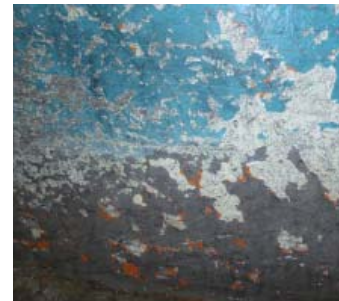
Detail of soiling and flaking paint near ground at tunnel.
