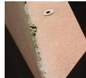
Detail of biological growth at weathering steel.
