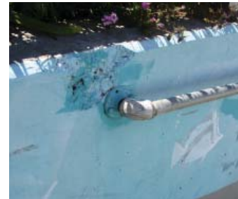
Detail of concrete spall at outdoor wall. Also note railing.
