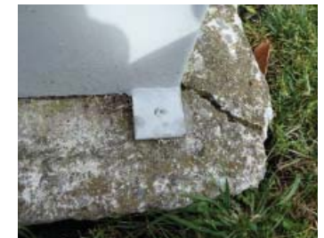
Detail of damage at concrete pad.
