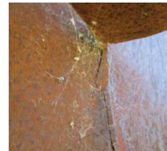
Detail of structural crack at front side (reverse side sim.)
