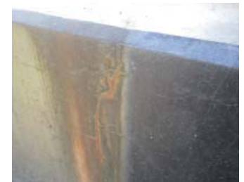
Detail of soiling and ferrous stains at base.
