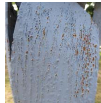
Detail of paint loss and corrosion at back of leg.
