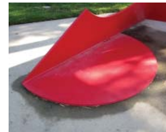
View of base plate. Note overall soiling, debris and surface water.
