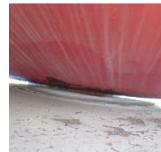
Detail of welded connection at base of tubular grid. Note heavy corrosion and staining/drip marks.
