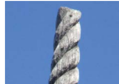
Detail of weathering at top of pole.
