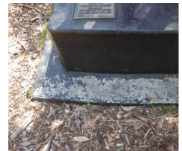
Detail of paint loss at the concrete pad.
