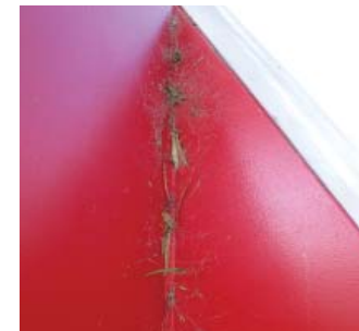
Detail of debris and insect nests at vertical joint.
