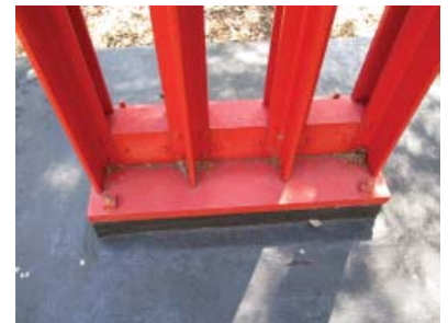
Detail of anchorage to plinth. Note soiling/ debris.
