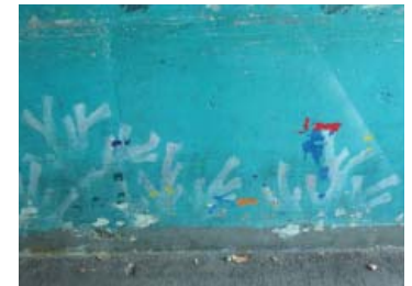
Detail of soiling and flaking at tunnel. Note primary colors below.
