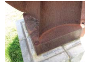
View of base. Note soiling, bio growth and guano.
