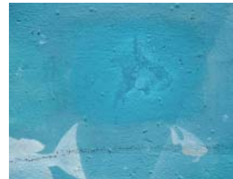
Detail of overpainting at tunnel wall.
