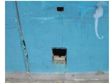
Detail of outdoor wall. Note missing grilles and deteriorated expansion joint
