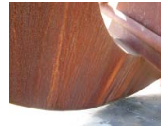
Detail of surface runoff stains at weathering steel.
