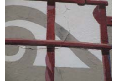
Detail of paint cracking at window grate.
