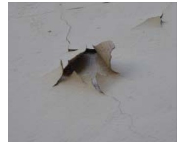
Detail of flaking and cracking paint at stucco wall.
