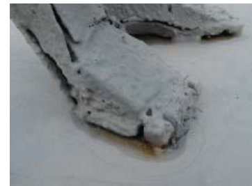
View of top of podium and feet. Note surface water, tide lines, and corrosion at welds.
