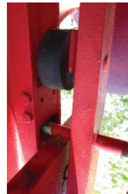
Detail of rubber stop and paint loss at pivot point.
