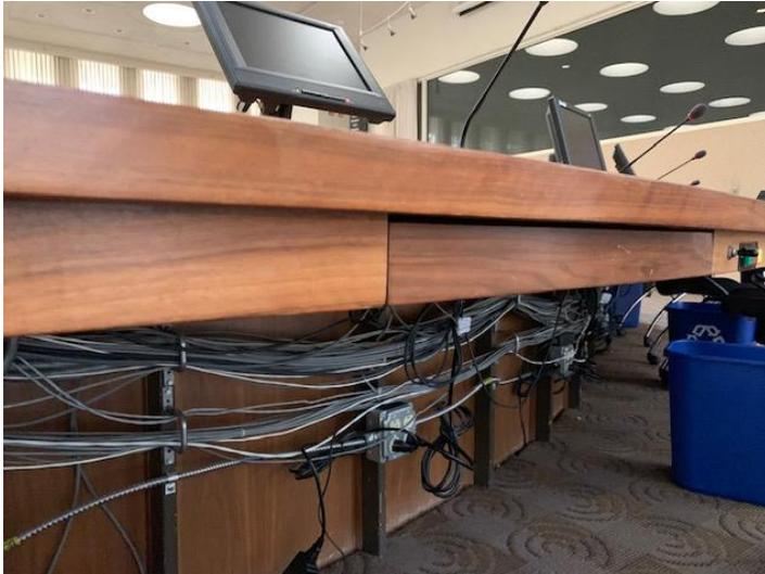
Figure 4 – Legacy wiring underneath the dais is a fire hazard to meeting members.
