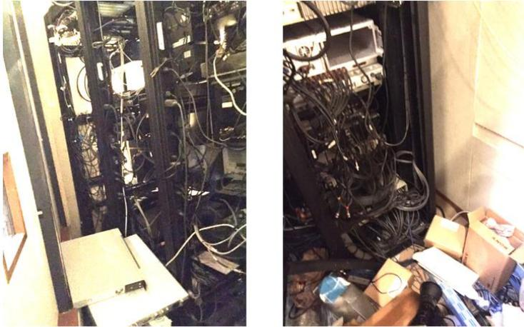
Figure 1 – The existing equipment’s cables and wiring are cumbersome and difficult to work with.
