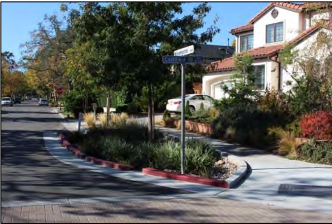
Southgate neighborhood bioretention planter
