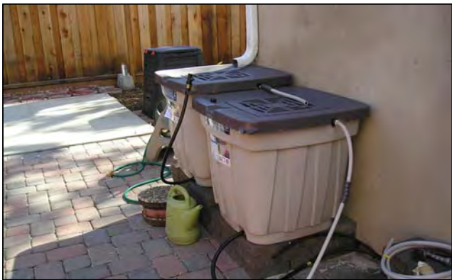
Rain Barrel Installation
