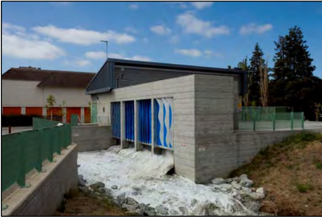
San Francisquito Creek Pump Station
