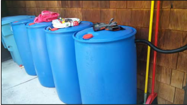
Rain Barrel Installation
