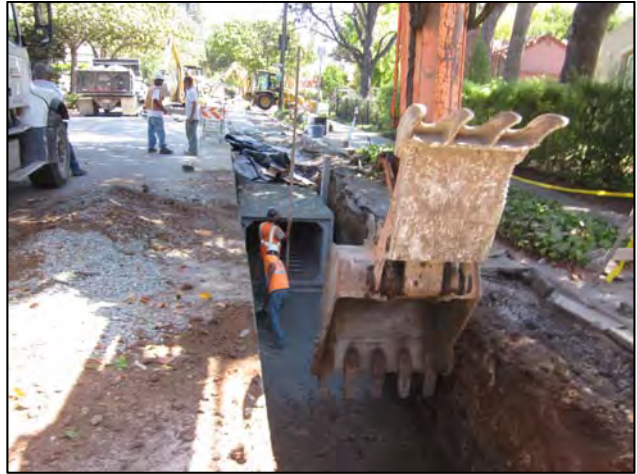
Channing Avenue box culvert
