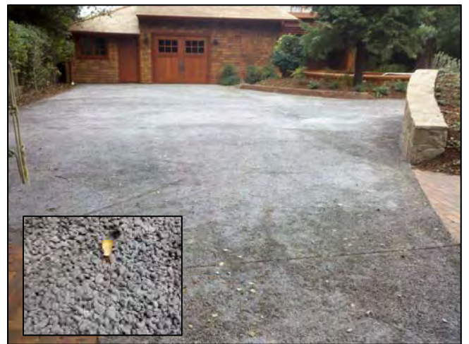
Pervious Concrete Driveway
