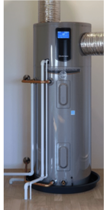
120 volt/15amp hot water heaters
