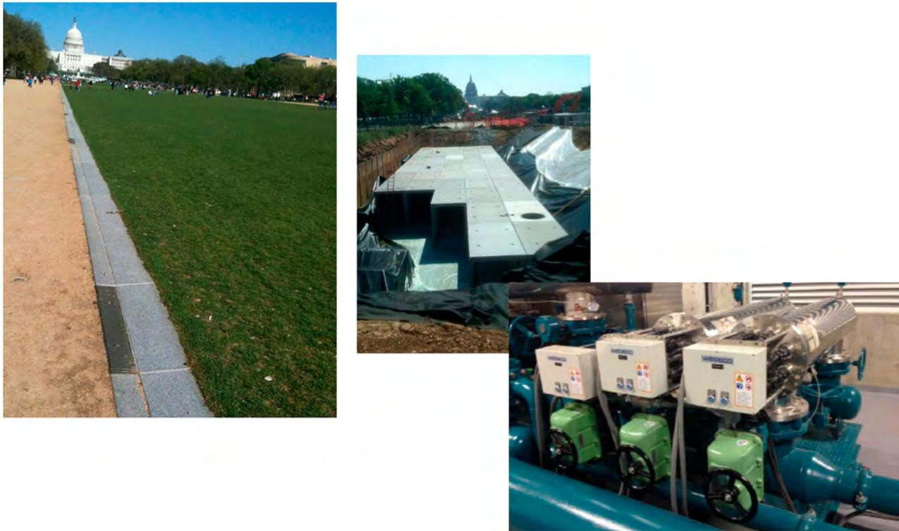
**Figure 1.** National Park Service constructed large stormwater cisterns under the National Mall for turf irrigation (center photo). Stormwater is processed through microscreens and ultraviolet light disinfection (right photo). On-site stormwater use is attractive where rainfall is more uniform throughout the year. (Right and left photos by the authors, center photo National Park Service).
