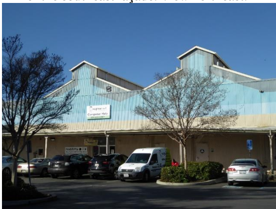
Figure 9. A pair of monitor roofs dominate the middle section of the southeast façade. View southwest.
