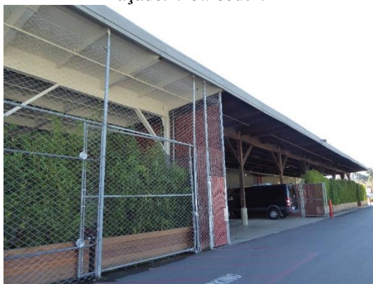
Figure 32. Wood post-and-beam construction under the awning at the south end of the northeast façade. View south.
