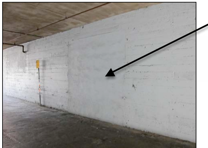
Figure 14. View along alley showing north wall of 451 Florence Street and the bank teller window infilled (arrow).
