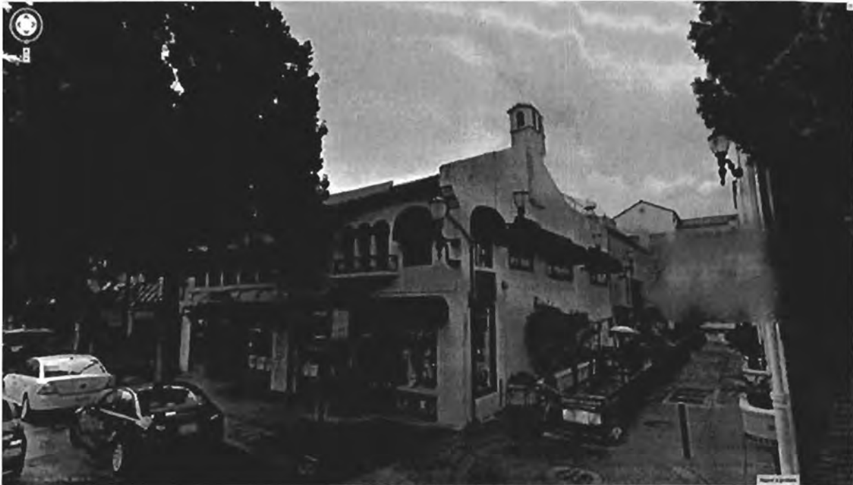
Building Prior to Renovations
