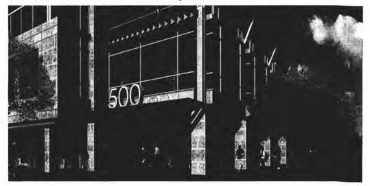
b) Retail Arcade: To ground the building, and make the retail arcade warm and inviting we propose transitioning the standard public sidewalk concrete with a dark grey band to land the columns, and then a medium grey paver in the arcade. This pallet of pavers is used throughout the project. The aluminum sunshade / light shelf is also the signage support. Please refer to sign program pages for those images.
