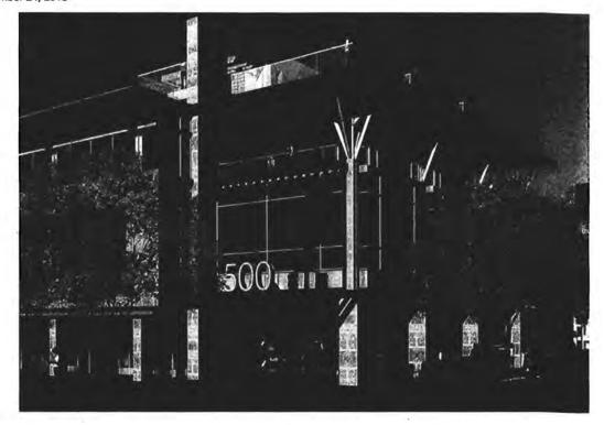
d) The tree brackets have changed significantly. They had been heavy, paired metal members trying to mimic wood. Now they are treated as steel and are lighter and more delicate, and have been recalled on the breezeway side of the building as well.
