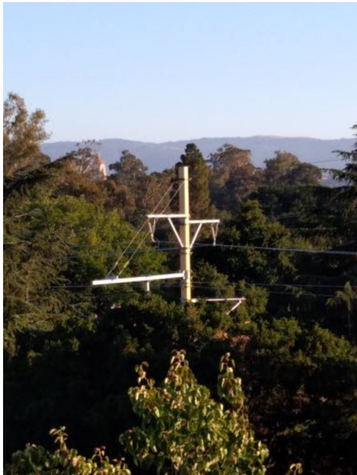
Figure 4, Pole projecting above the tree tops.
